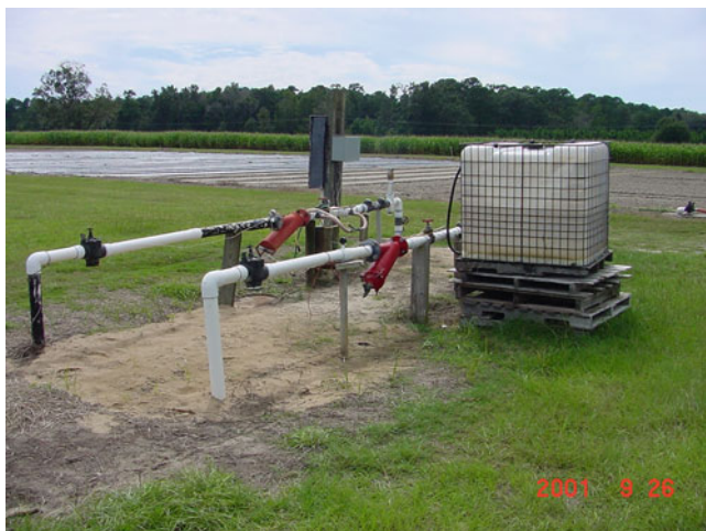
Fig. 4 Liquid fertilizer tank mounted on a pallet, containing liquid 8-0-8 and used for the injection of N and K into the two drip irrigation systems using Mazzi injectors. Note on each system (from right to left), the back flow prevention device, the injection port, the pressure gage, the screen filters (in red), and the solenoid valve (in black; photo credit: Robert Hochmuth)
