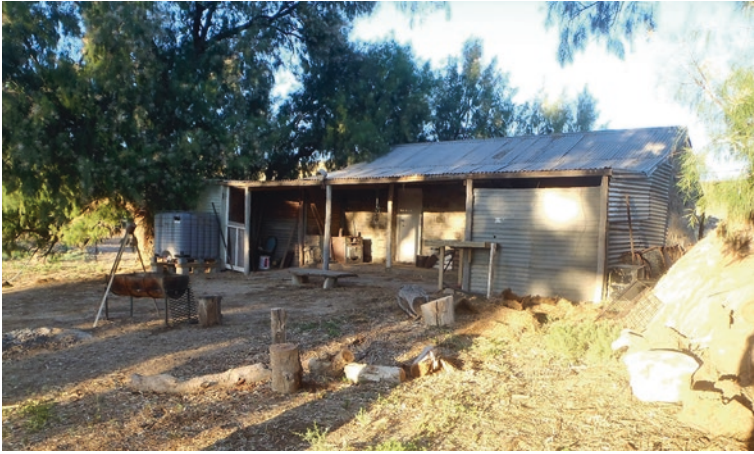
Fig. 26.1 Douglas Hut, Yankaninna, Flinders Ranges, South Australia
