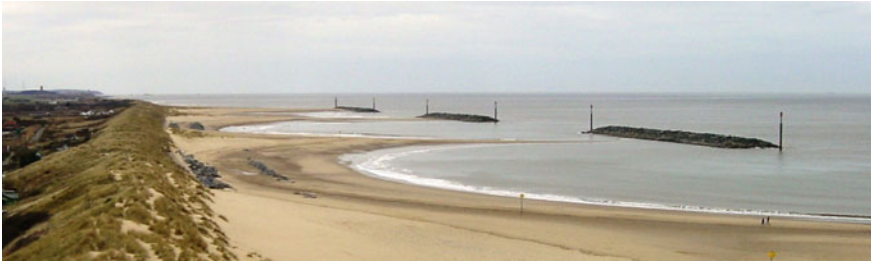
Fig. 7 Beach response to detached breakwaters at Sea Palling, UK. Accretion of the shoreline towards the structure can be observed
