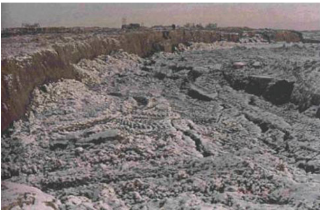
Fig. 6 Swiniec landslide below level +415, Dec. 1994
