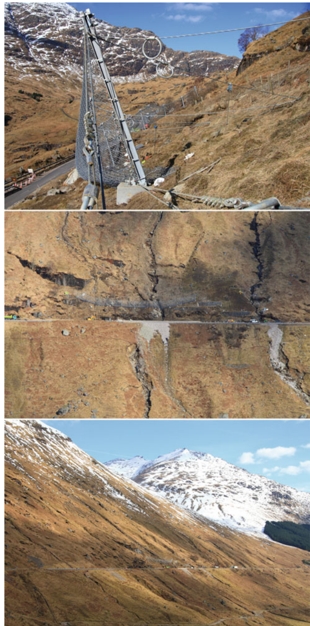
Fig. 3 Debris flow barriers
