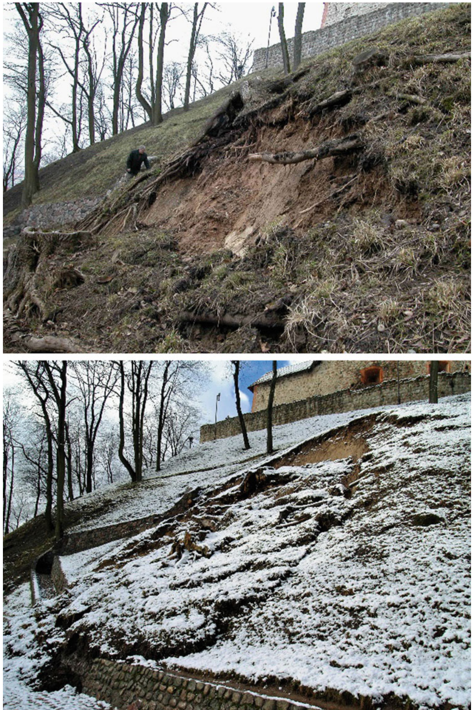
Fig. 5 Landslide in the eastern slope of Gediminas Hill formed in March, 2004 (above) and reactivated in March, 2008 (photos by Vidas Mikulėnas)
