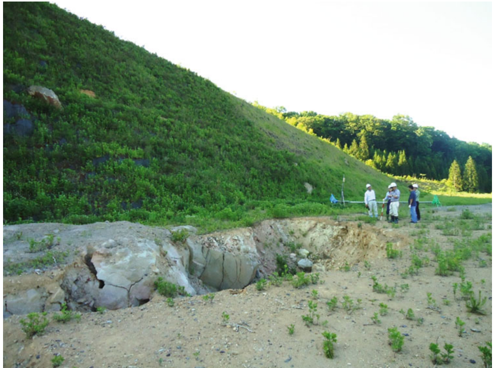
Fig. 2 Continuous cracks at upper part of the head scarp, monitored by the extensometers
