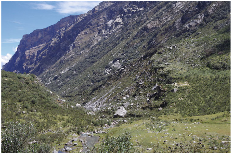
Fig. 2 Example of debris cone dam of Lake Yircacocha which failed on 13th December 1941 as a result of a flood wave from upstream situated Lake Palcacocha. Breach width is about 150 m and breach depth >25 m. Former lake water level is visible in the right part of the figure
