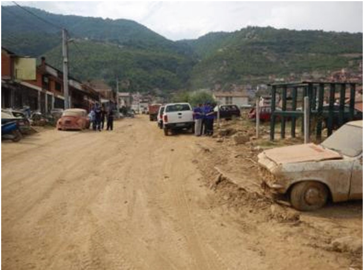
Fig. 7 Village road in Mala Recica was covered with mud
