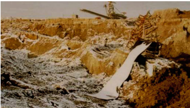
Fig. 5 Swiniec landslide view from level +415, Dec. 1994
