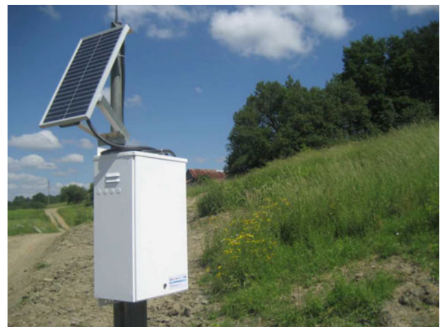
Fig. 14 Automatic monitoring station (Bednarczyk 2014)
