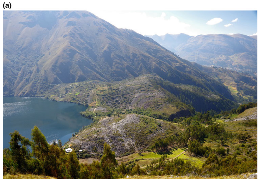
Fig. 5 Part a shows rockslide originating from right bank damming Lake Purhuay; part b shows upstream view on deeply eroded dam
