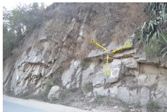
Fig. 2 Field Photograph and stereo plot of rock slope no. 21
