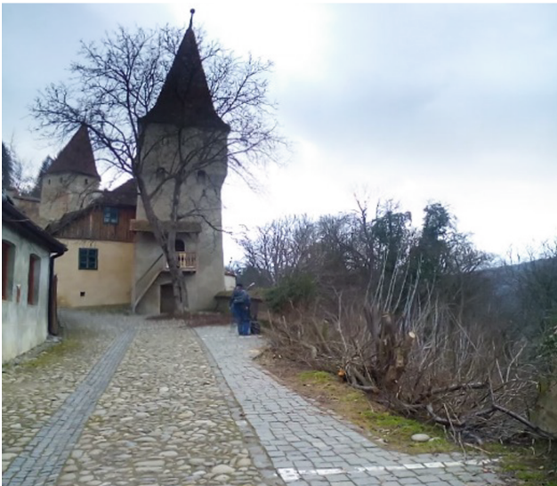
Photo 1 Tailor Tower and damaged wall (a 2006; b 2016)
