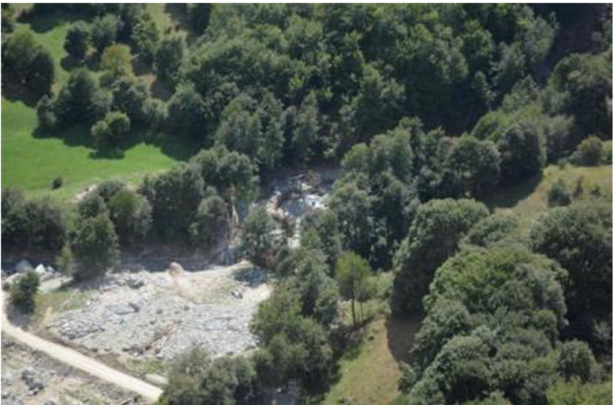
Fig. 5 The road between Sipkovic and Brodec was completely covered with debris flow material
