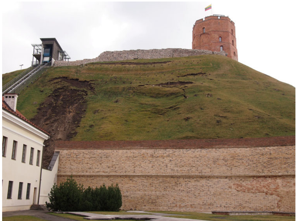
Fig. 7 Slope failures of different shape and development on the representative slope of Gediminas's Hill in March 2016 (photo by Vidas Mikulėnas)
