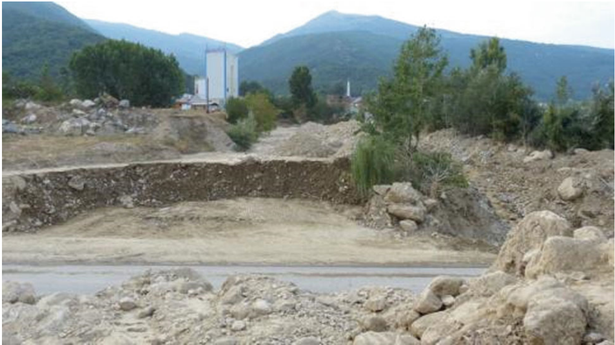
Fig. 6 Debris flow deposits in the Poroj
