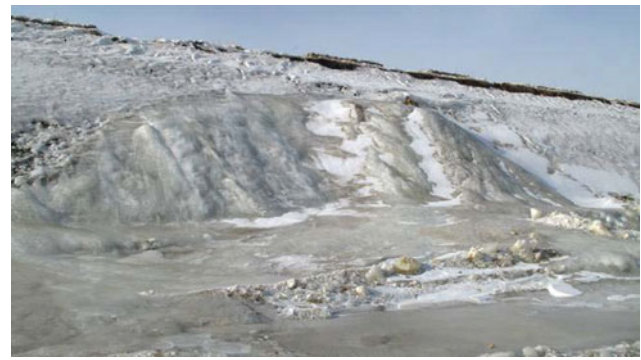
Fig. 9 Icing on the cut slope during the freezing period (February 2010) as well as location of this icing point
