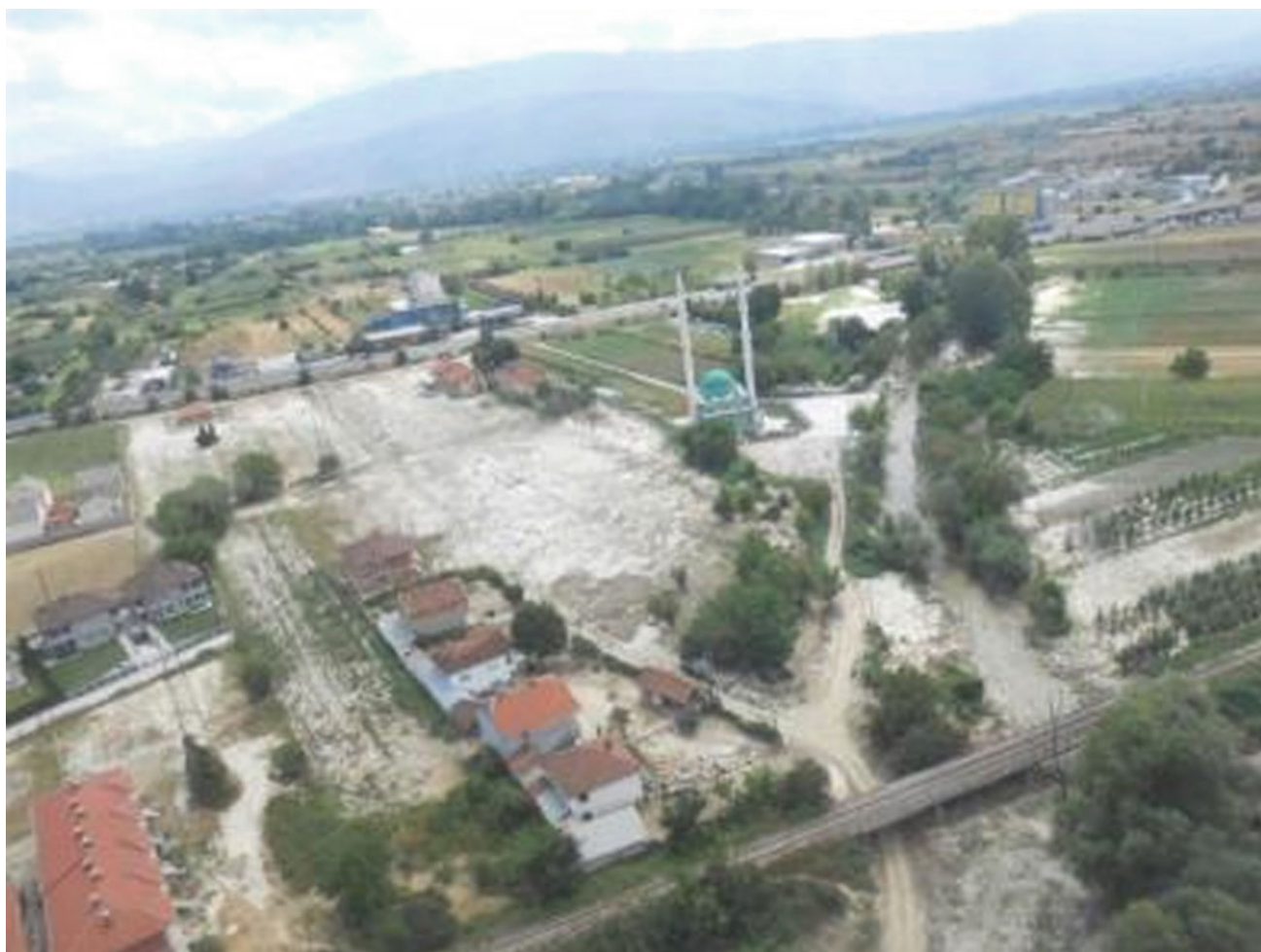
Fig. 11 Flooded area in the city Tetovo
