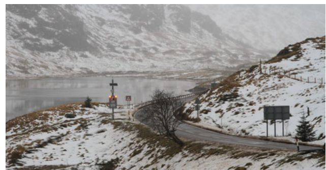
Fig. 2 Wig-wag signs offer both a geographical (non-temporal) and a temporal, or early-, warning
