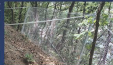
Debris flow barrier and rockfall barrier that we installed in Seoul Korea.
