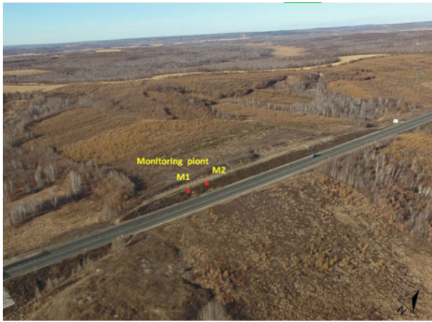
Fig. 3 Topography of K162 cutting slope of the Highway (40 m wide)
