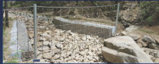
Debris flow barrier and rockfall barrier that we installed in Seoul Korea.
