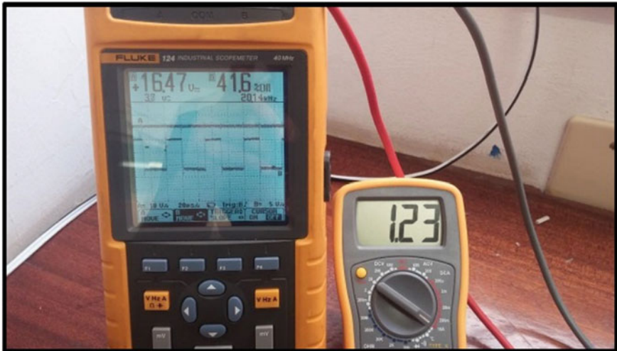
Fig. 22 Solar panel voltage and current under partial cloudy condition
