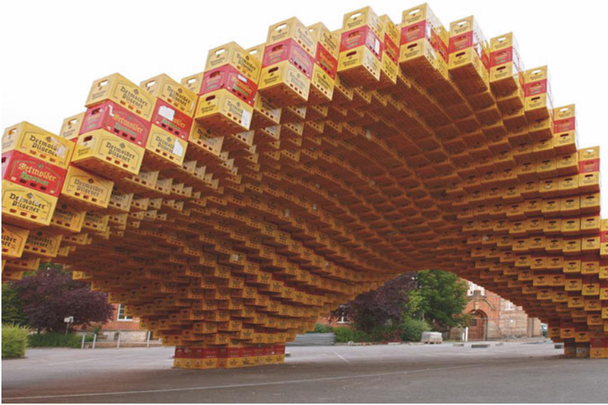
Fig. 8 View of the structure with a 15 m span and a total height of 5 m
