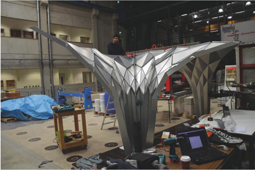
Fig. 8 Building the 1:1 mock-up
