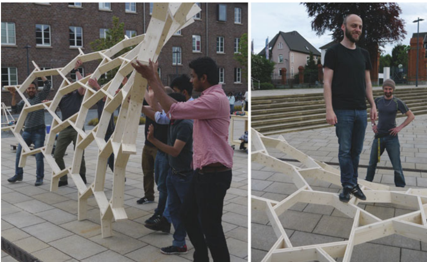
Fig. 10 Positioning and testing the reciprocal structure
