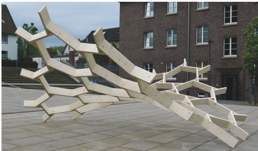
Fig. 11 Reciprocal structure on the Campus Emile in Detmold
