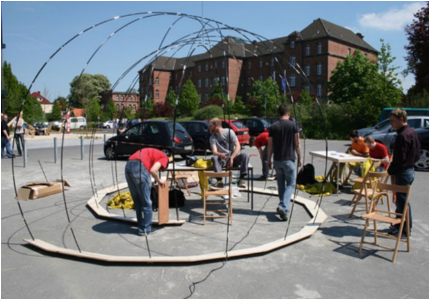
Fig. 6 Assembly of the arcs on the University campus Emilie in Detmold
