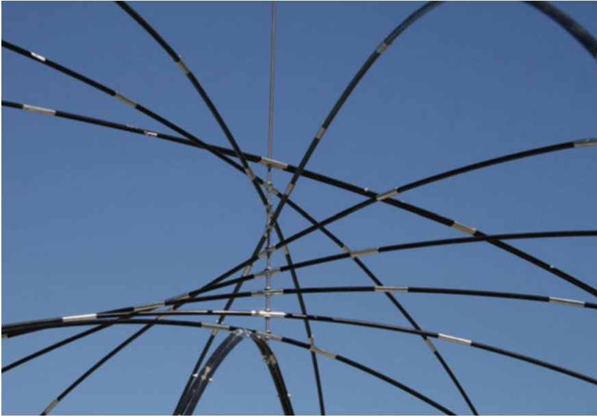
Fig. 7 Central connection detail
