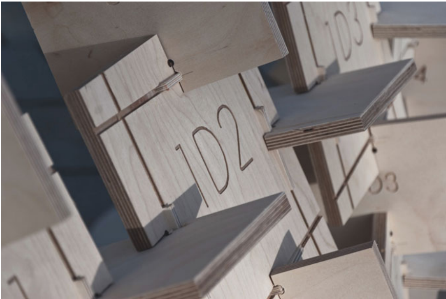
Fig. 15 SunSys connection detail
