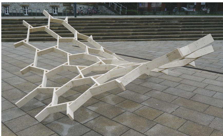
Fig. 12 Reciprocal structure on the Campus Emile in Detmold
