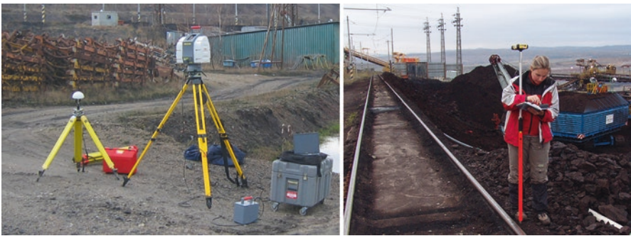
Fig. 4.24 Mapping the surface coal mine with 3D laser scanner HDS3000 (on the left side) and GPS (on the right side)
