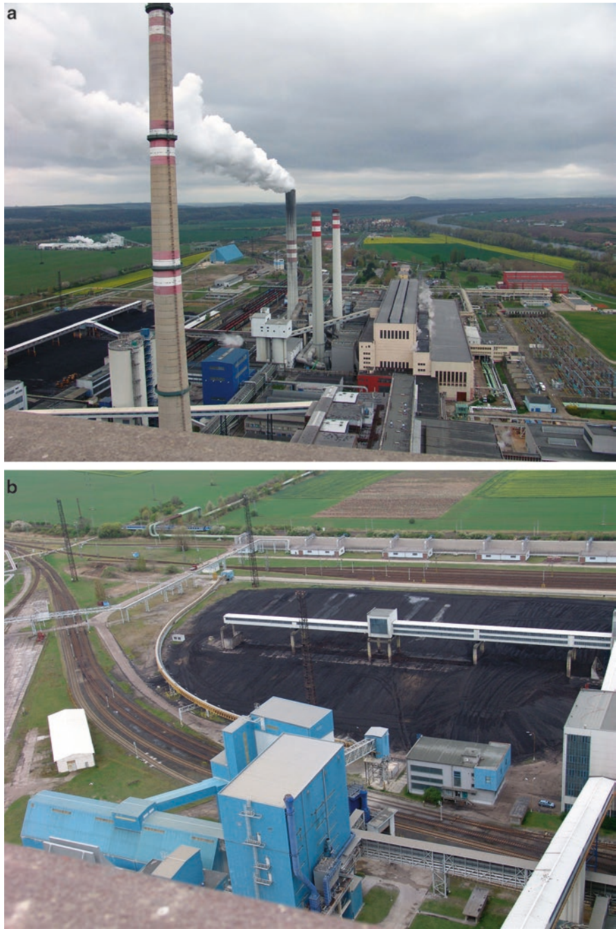
Fig. 4.3 (a) Fossil-fueled power station for production of electricity and for central heating of neighbor residential sites. (b) Temporary coal storage of the fossil fueled power station
