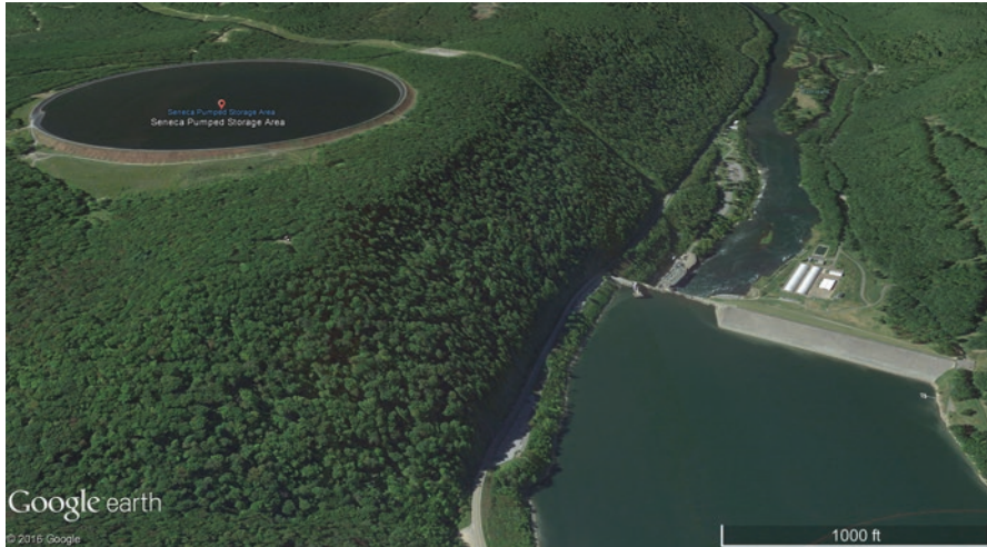
Fig. 10.4 The Seneca pumped-storage generating station in northwest Pennsylvania takes advantage of the local topographical conditions by filling a reservoir at a higher elevation than the dam below. Source: Google Earth, 2016
