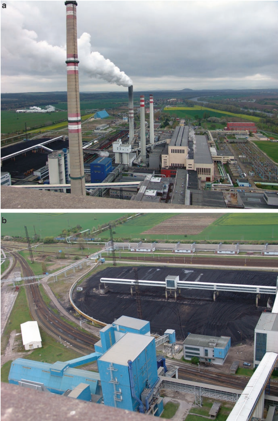
Fig. 4.3 (a) Fossil-fueled power station for production of electricity and for central heating of neighbor residential sites. (b) Temporary coal storage of the fossil fueled power station
