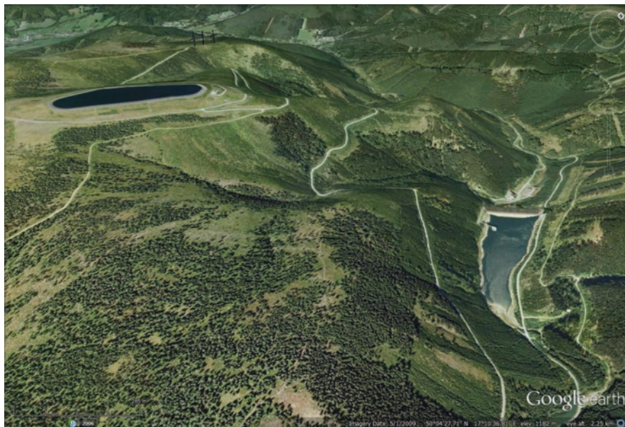
Fig. 5.8 A view on lower and upper reservoir of a pumped-storage plant. Source: Google Earth, 2016
