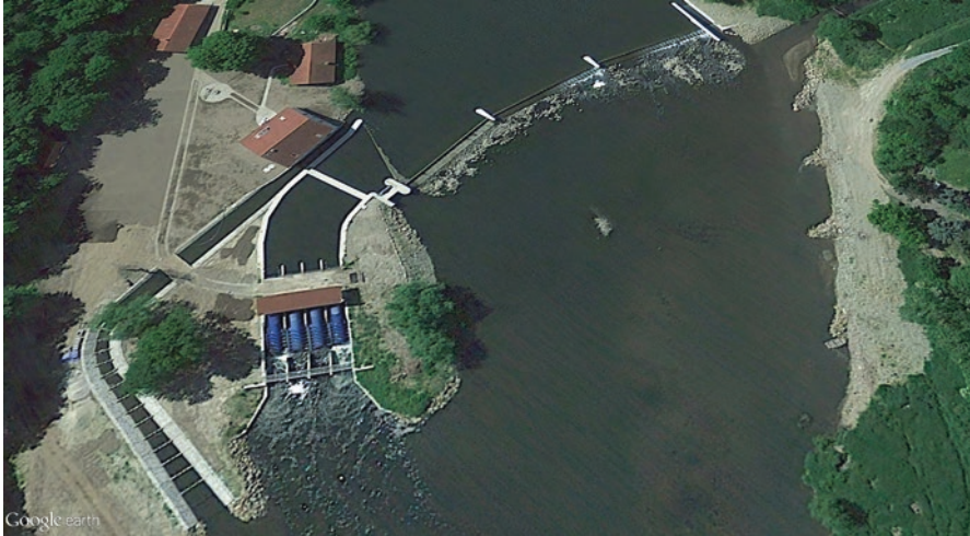
Fig. 5.11 Screw turbines at a small hydropower complemented by a weir and a fish ladder. This construction is considered to be friendly to aquatic wildlife (labeled as “fish friendly”)
