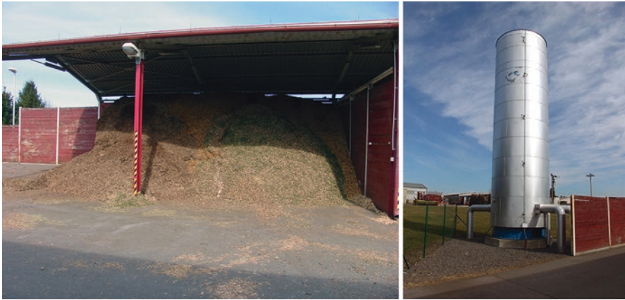
Fig. 8.3 The use of biomass (wood chips) in a heating systems and a buffer tank for thermal stores (on the right side )
