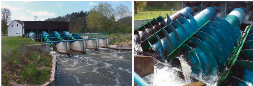
Fig. 5.10 A screw turbine (reverse Archimedes’ screw): the hydropower plant and a detailed view on the screws
