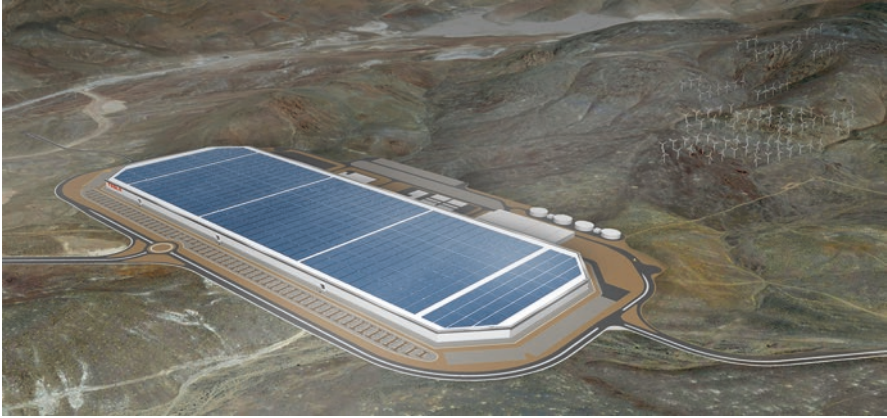
Fig. 10.7 Tesla Gigafactory (planned annual battery production capacity of 35 GWh). Source: https://www.tesla.com/ , 2016
