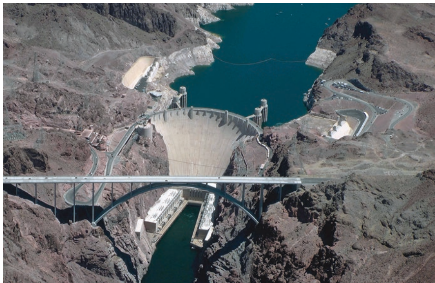
Fig. 5.1 Hoover Dam, a concrete arch-gravity dam in the Black Canyon of the Colorado River in the United States. It was constructed between 1931 and 1936, the height of the dam is 221.4 m, and the installed power capacity is 2080 MW. Hoover Dam impounds Lake Mead, the largest reservoir in the United States by the total capacity 35,200 km 3
