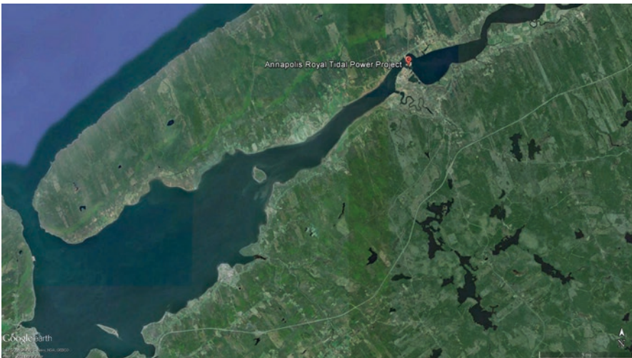
Fig. 5.13 The Annapolis Tidal Power Plant (20 MW) with a daily output of roughly 80–100 MWh, depending on the tides. Source: Google Earth, 2016
