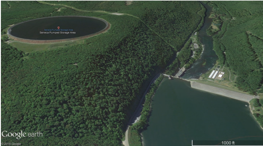
Fig. 10.4 The Seneca pumped-storage generating station in northwest Pennsylvania takes advantage of the local topographical conditions by filling a reservoir at a higher elevation than the dam below. Source: Google Earth, 2016
