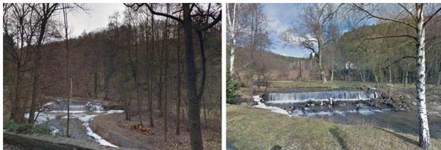
Fig. 5.23 Examples of two weirs on a downstream part of the basin. Source: Google Earth, 2016
