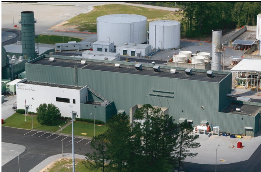
Fig. 10.5 Compressed air energy storage at McIntosh power plant in Alabama. Source: PowerSouth Energy Cooperative, A Touchstone Energy Cooperative, 2016, http://www.powersouth.com
