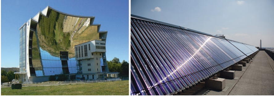
Fig. 7.12 A solar tower for high temperatures and heating of water (on the right side ). Source: www.pixabay.com , 2016
