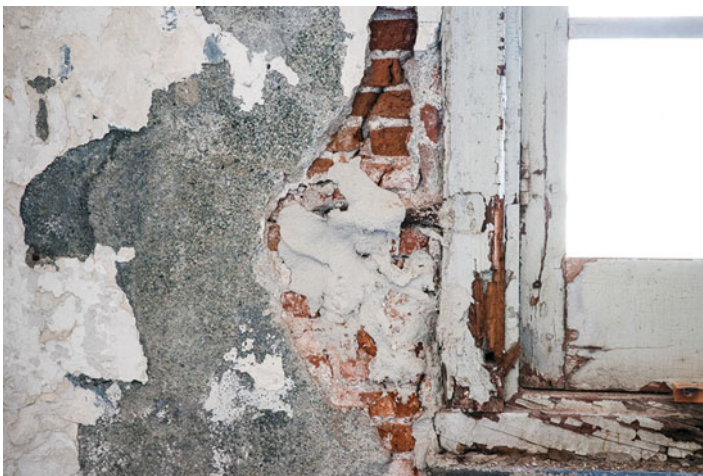
Fig. 6.36 The fixed frame, devoid of sub-frame, is anchored onto the jamb through metal clamps
