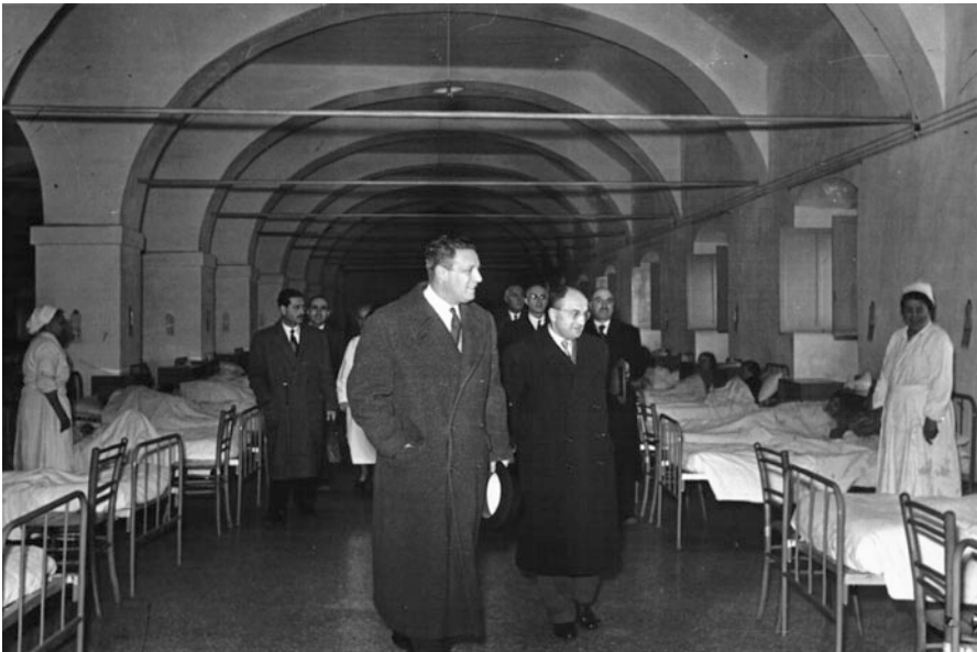
Fig. 6.13 Brick arches between pillars and outer wall; the horizontal thrust is contrasted by the insertion of iron chains (AIB, folder 18)
