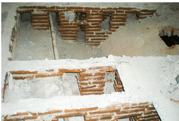
Fig. 6.11 Lightened brick walls placed at the extrados of a vault; note that the wheel base is such as to enable a thin slab of stone (usually slate) to rest
