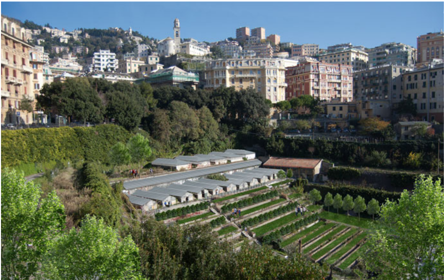
Fig. 8.10 Restoration of the greenhouses system with glass PV cells (photo-simulation) (Macchioni, E. (2016). Post-graduate in Architectural Heritage and Landscape, University of Genoa)
