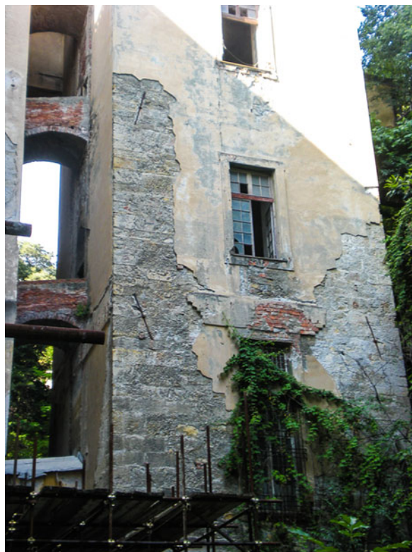
Fig. 6.2 In the lavatory towers, square blocks have been used
