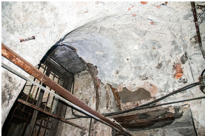
Fig. 6.20 Slate plate in the lower part of a wattle vault
