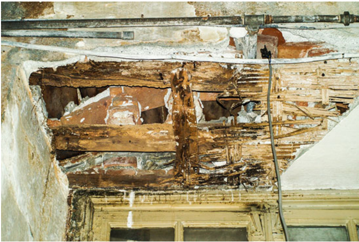
Fig. 6.40 Lintel of a window covered with plastered wattle
