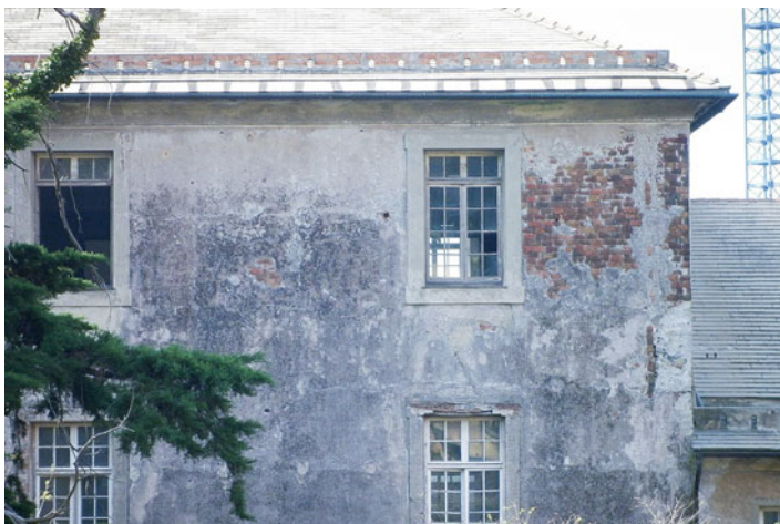
Fig. 6.5 Solid brick masonry on the top northern tower floor
