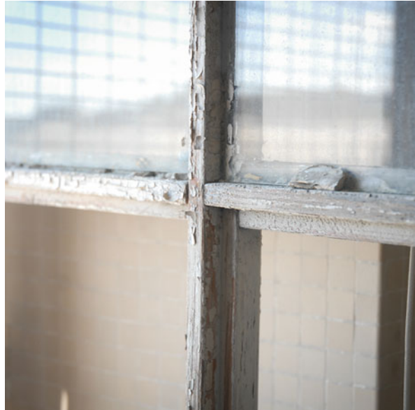
Fig. 6.37 The windows of the Albergo dei Poveri complex are divided into squares through slender glazing straight edges
