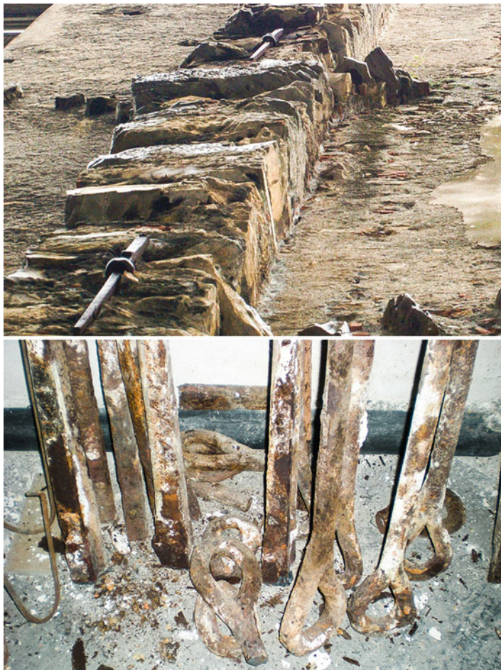
Fig. 6.7 End-plate stakes in correspondence of a spine wall (at the top ). Metal chains removed at the time of the recent interventions for the redevelopment of the complex; quite visible are the eyelets built at the ends where the end-plate stake would be inserted (at the bottom )
