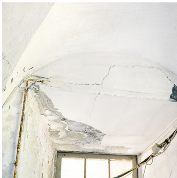
Fig. 6.19 Soffit of an opening made with slate plates nailed to a supporting wooden structure
