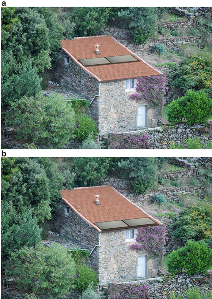
Fig. 9.8 (a, b, c, d) Schiara, Italy, UNESCO site. Different type of arrangement of solar panels have incidence of the visual perception of the roof
