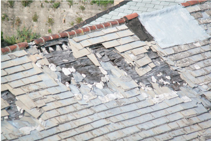
Fig. 6.21 Slate roofing laid on a wooden plank
