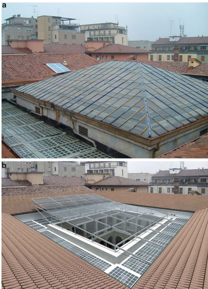
Fig. 9.1 (a, b) The new covering system of Banca Monte dei Paschi di Siena in the historical centre of Mantova (picture b), Italy (arch. Franco Biondi), compared with the state before the intervention (picture a)
