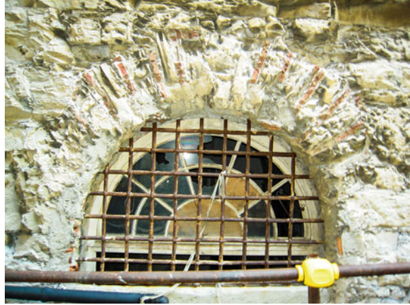
Fig. 6.12 Stone-and-brick arch in a wall to derive the gate of the window
