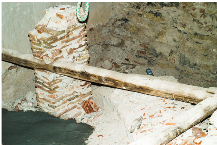
Fig. 6.10 Reinforcement ribs in a brick vault
