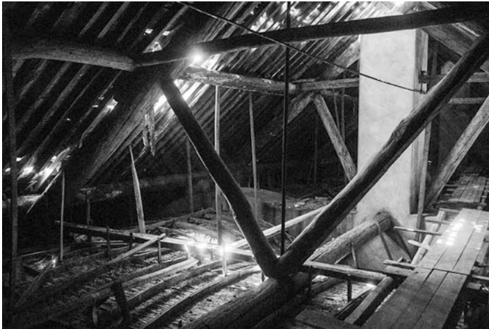
Fig. 6.26 Roofing structure of the north-west wing. The horizontal beams rest on wooden pillars, struts, and frames
