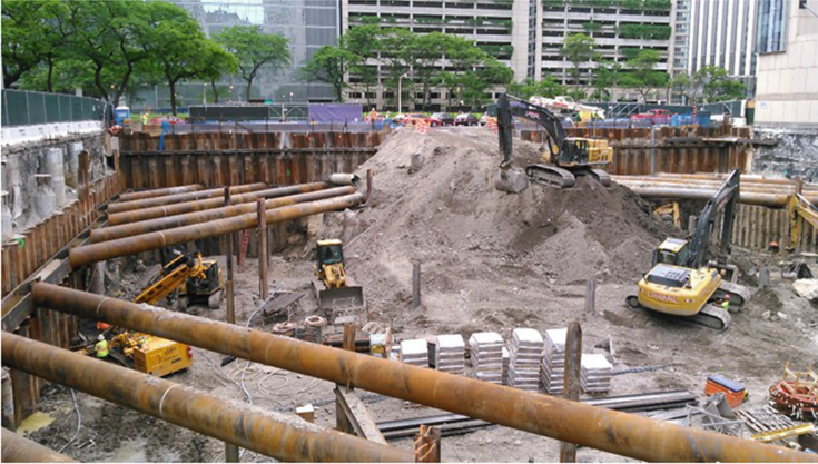
Fig. 5. Site activities during task 10
