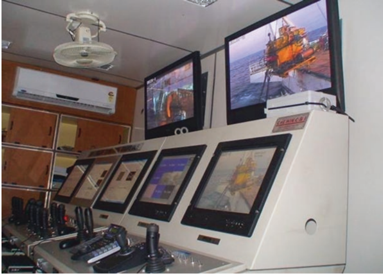
Fig. 10.29 View of onboard control room
