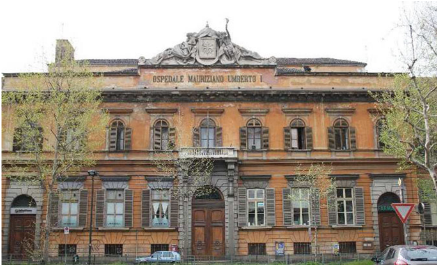
Fig. 1 The Mauriziano hospital in Turin, Italy
