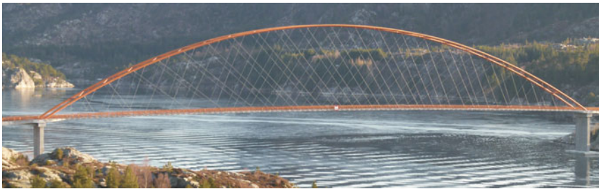
Fig. 3 The brandanger bridge
