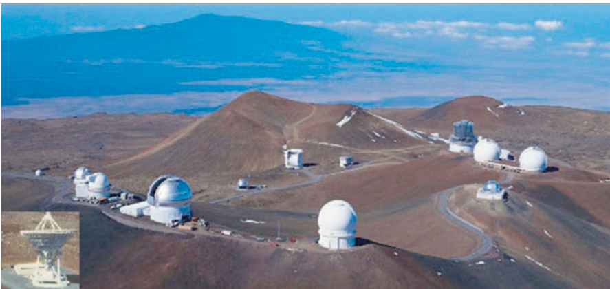
Fig. 8.3 Aerial view of Mauna Kea Observatory (Institute for Astronomy, University of Hawaii)
