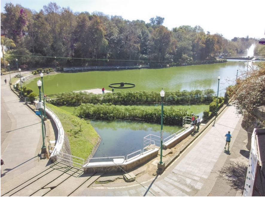
Fig. 10.1 Two large Floating Wetlands have been established as an efficient aquatic phytobarrier or phytofilter at the entrance of Lake 1 in the Lakes System known as “El Dique” en Xalapa, Veracruz, México [22]
