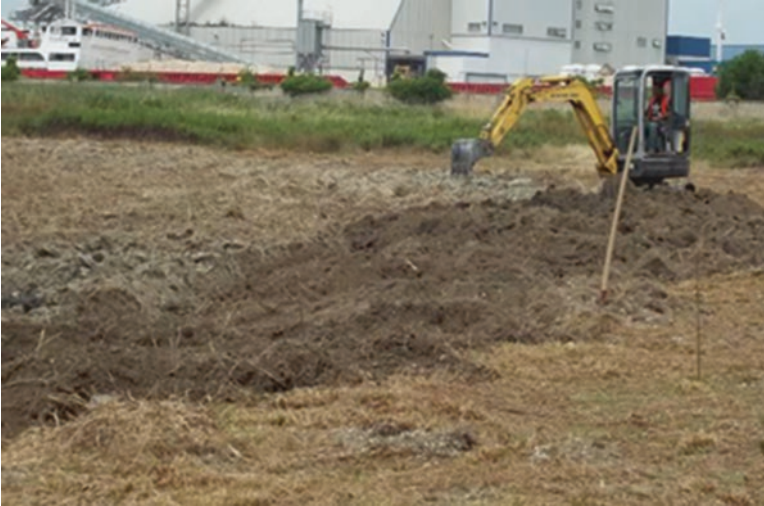
Fig. 3.5 Moving top-soil with excavator
