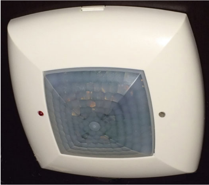
Fig. 2 Two channel presence sensors used for the stationary assistance subsystem (Theben Office™)—1st channel for (local) automatic room lighting control, 2nd channel for presence signaling to assistance system
