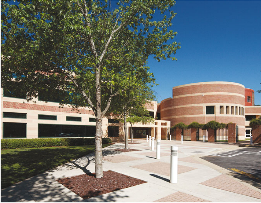
Fig. 1 The Biotechnology Center's headquarters site in the Research Triangle Park houses staff offices as well as a conference center with meeting rooms of different sizes, a 170-seat auditorium, and open space to accommodate vendor shows or poster sessions. Additional office space can be rented by start-up companies ( Source NCBiotech/Jim Sink)
