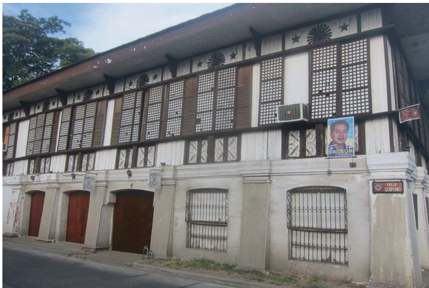
Fig. 14.6 Syquia Mansion, former house of President Elpidio Quirino in Vigan, Ilocos Sur (April 2016) The lower-level stone structure is clearly visible, as is the upper level lighter wood frame. The windows on the upper level give to the volador running on the entire side of the main room. The largest lower opening is the zaguan. The house contains an inner garden on the top level. An exterior air conditioning unit is a recent concession to “modernity”. As the home a former president, this house is now a museum within a city which is also a UNESCO heritage town
