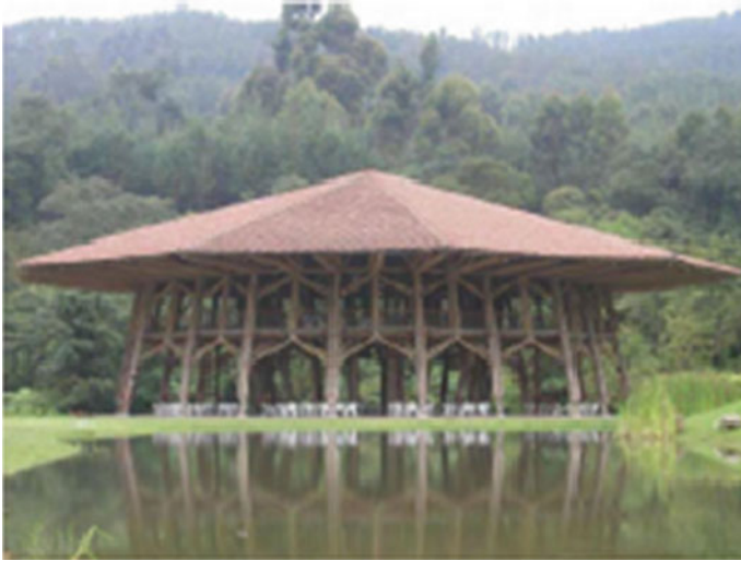
Fig. 9 Exterior view of the ZERI Pavilion built in Manizales Colombia (Salas 2006)
