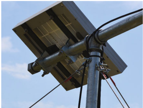
Fig. 9 The solar panel fitting
