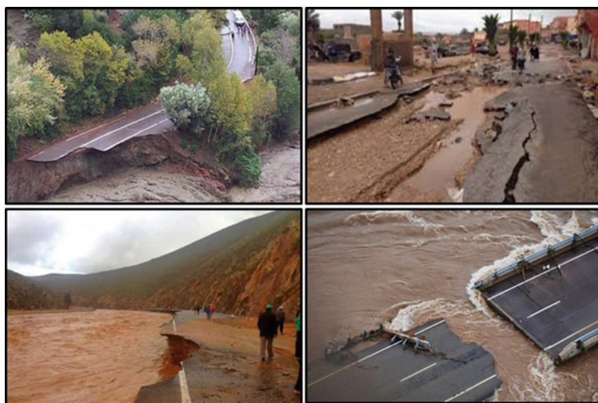
Fig. 2 Destruction of several roads and bridges' infrastructure in Guelmim city region in December 2014 (Photos from the web)
