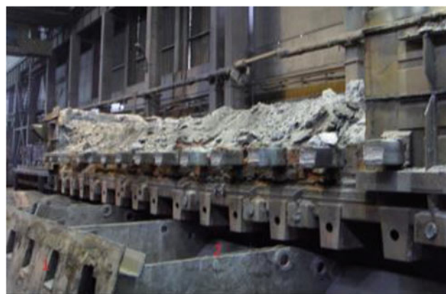
Fig. 1 Cell switched off for re-lining
