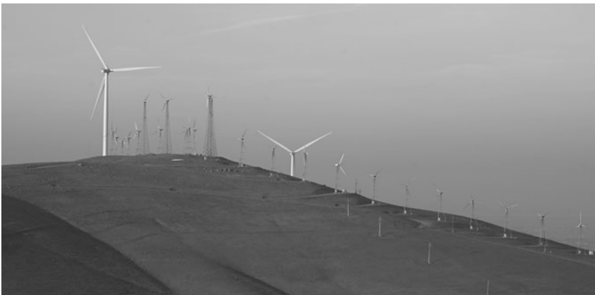
Fig. 2 In this example in the Altamont Pass WRA, California, all of the small wind turbines can be replaced by the single large turbine at the hill peak to achieve the same rated capacity, although the capacity factor would be increased 3- to 4-fold and the available space available for careful siting increased by a factor of >20
