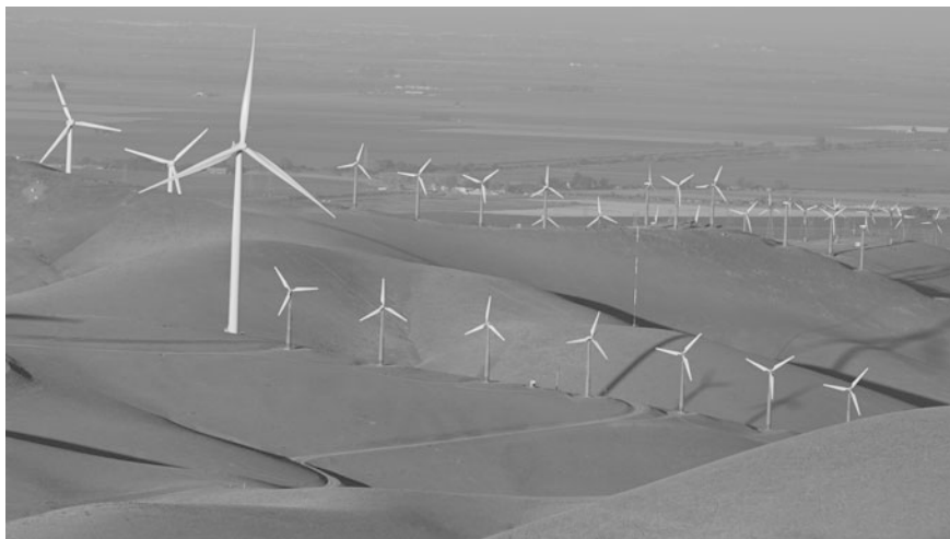
Fig. 3 In this example in the Altamont Pass WRA, California, a 2.3 MW turbine was installed next to 7 120-KW Bonus turbines descending along a ridgeline into a ravine where raptor collision risk is generally higher. Nineteen of the Bonus turbines can be replaced by a single 2.3-MW turbine
