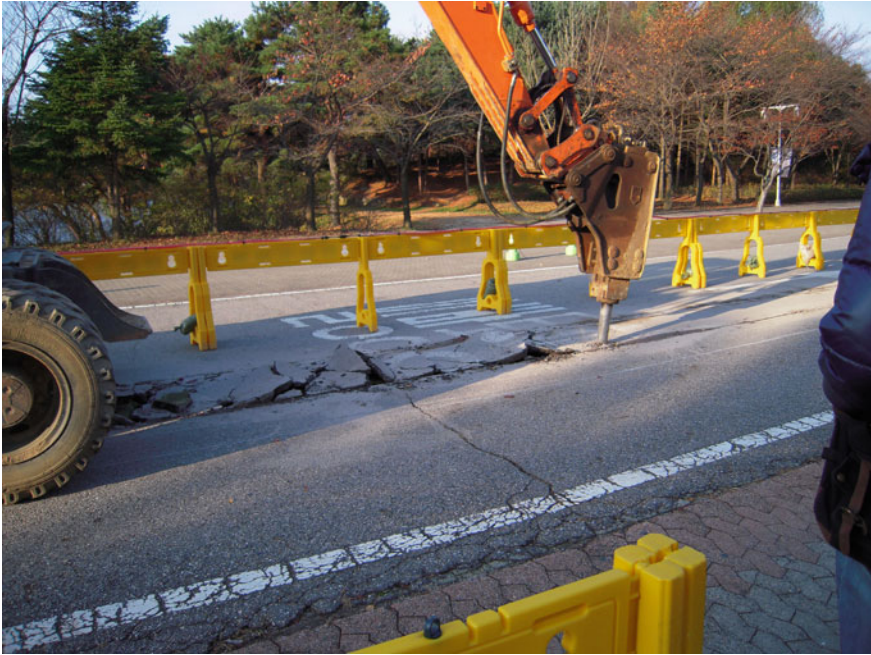
Fig. 11.5 Process for excavating existing road
