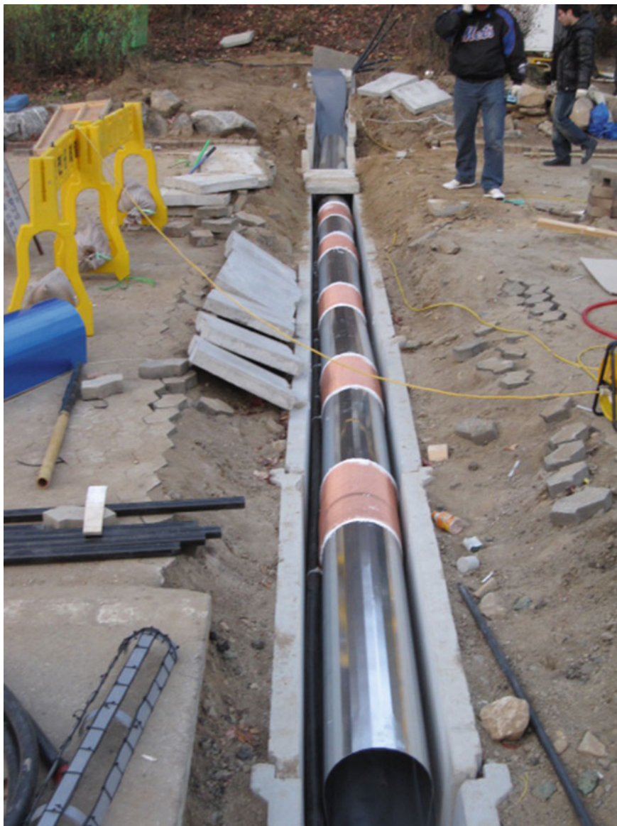
Fig. 11.8 EMF shielding work at regions in excess of EMF safety level
