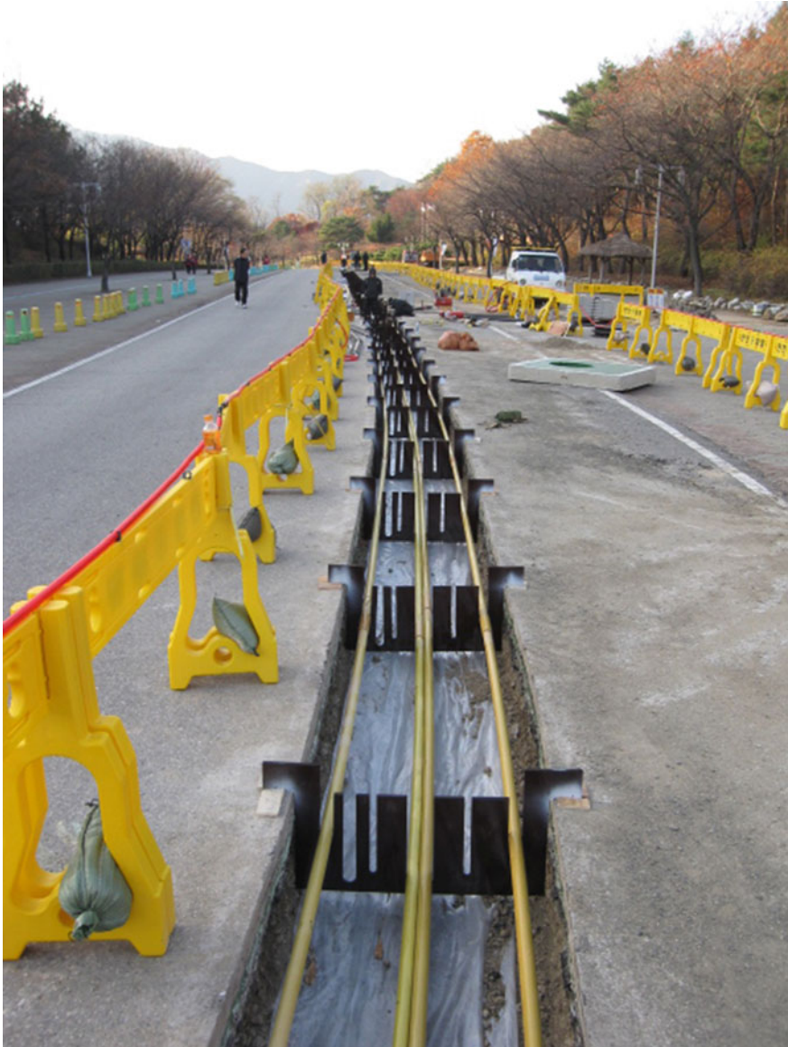
Fig. 11.6 Structure prepared to install power supply system
