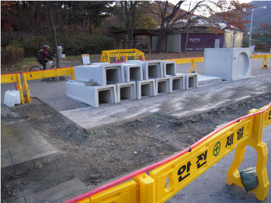
Fig. 11.4 Cutting work of selected road
