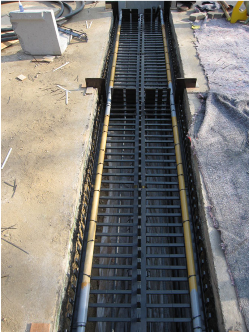
Fig. 11.7 Installation of the road embedded power supply system
