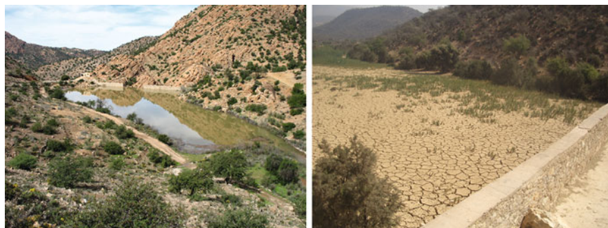
Fig. 12 Example of high and moderate dam's siltation: Assgherkiss dam with low siltation and Tildi dam completely silted
