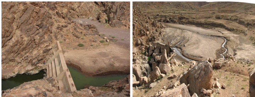
Fig. 14 Dam’s silting by bed load transport in high altitude: case of Adghigh and Talate dams
