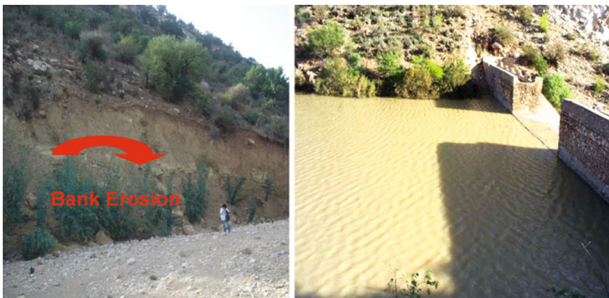
Fig. 13 Bank erosion and its consequence in Tildi dam. The turbid color of water reflects the eroded marl formation
