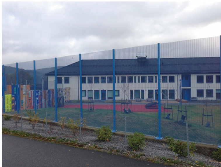
Fig. 13.1 The finished prison building
