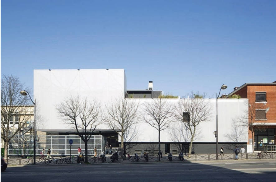
Source: Photography by: Michel Denancé. Recovered from: http://mx.archello.com/en/project/ecole-42
