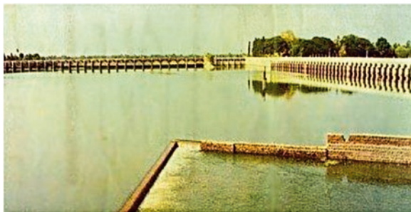
Pic 32 This oldest dam in the world, Grand Anicut (Kallanai), is located in Tamil Nadu built by the Chola King Karikalan in the first century AD. Source: http://www.tamilspider.com/resources/3363-Grand-Anicut-Kallanai-Tamilnadu.aspx
