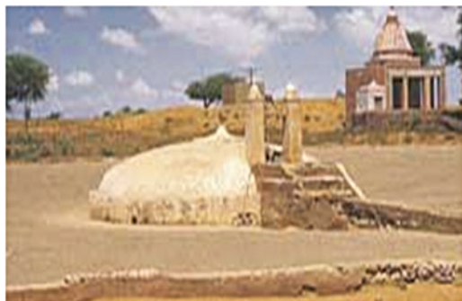
Pic 20 The picture is of a Kunda in the state of Rajasthan that is still in use. Source: http://www.esamskriti.com/essay-chapters/Traditional-Methods-of-Water-harvesting-and-applicability-2.aspx
