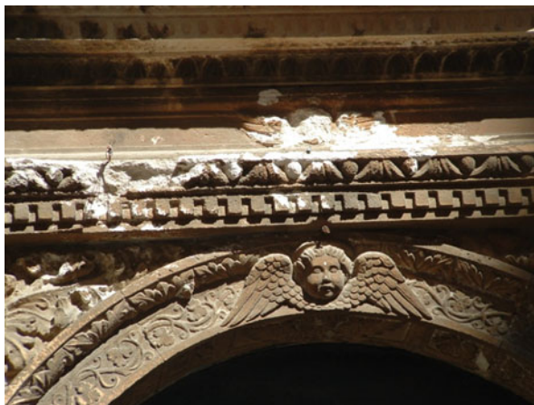
Fig. 3.12 Historical center of Dubrovnik: molded frame affected by the black crust
