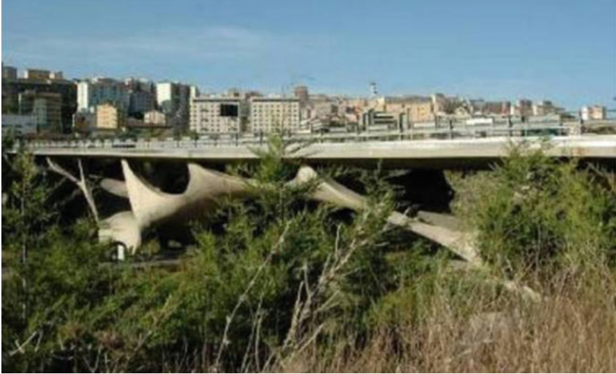
Fig. 25.2 Basento Viaduct in Potenza, detail of a span (Source: figure in Bavusi et al. 2011)
