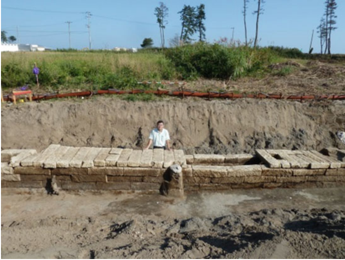
Fig. 27.8 The sewer system re-found by GPR survey
