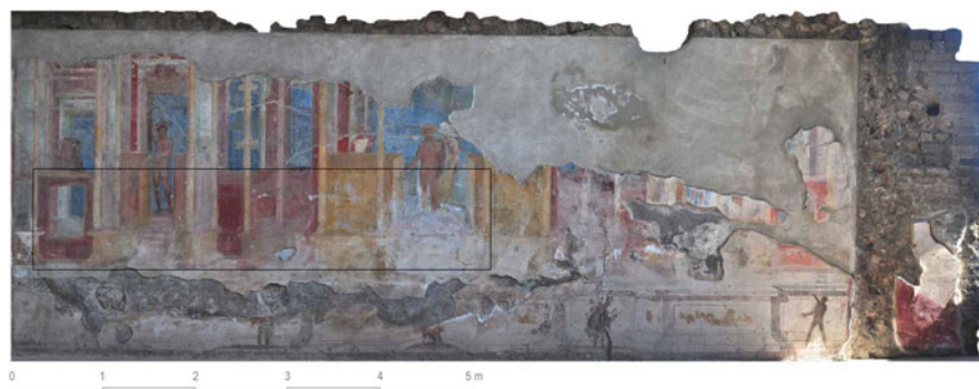
Fig. 29.13 The Gymnasium: Orthophotograph of the south wall painting. The black rectangular box denotes the area of fresco investigated by GPR
