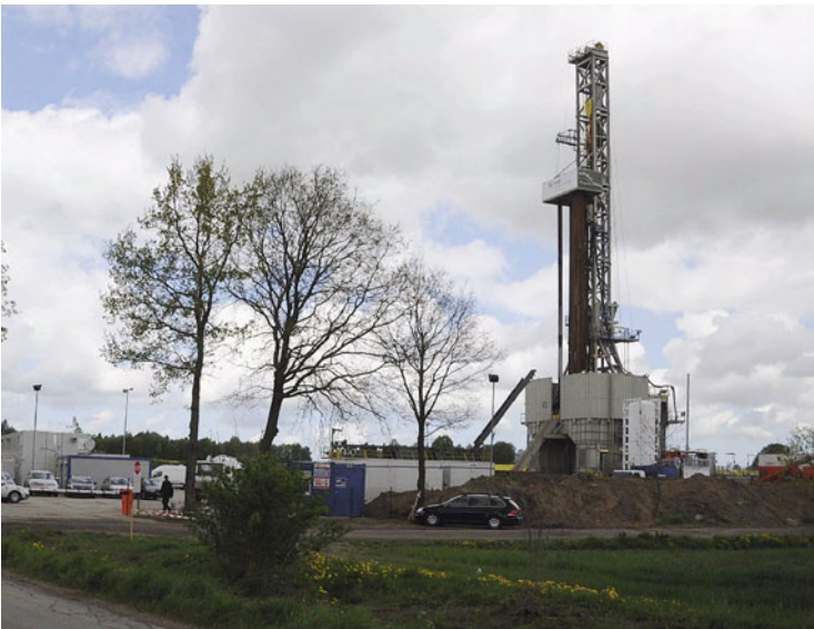
Fig. 2 Shale gas rig in Lebien, in northern Poland, where Lane Energy Poland company does test drilling ( http://www.mlive.com/business/mid-michigan/index.ssf/2011/06/is_growing_shale_gas_revolutio.html )
