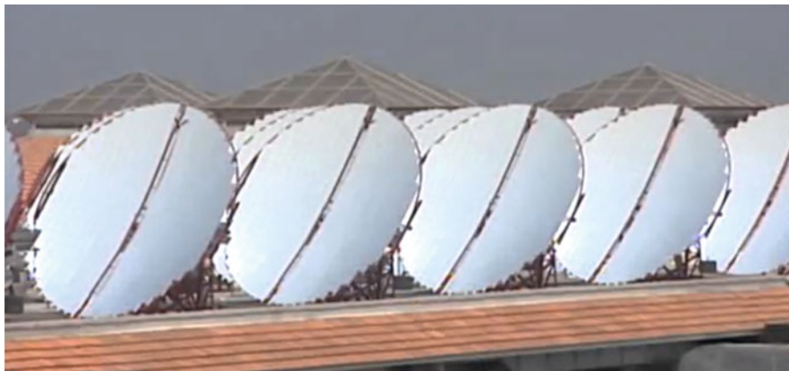
Fig. 17.6 World's largest solar cooking system in Shirdi which can cook for 100,000 people per day
