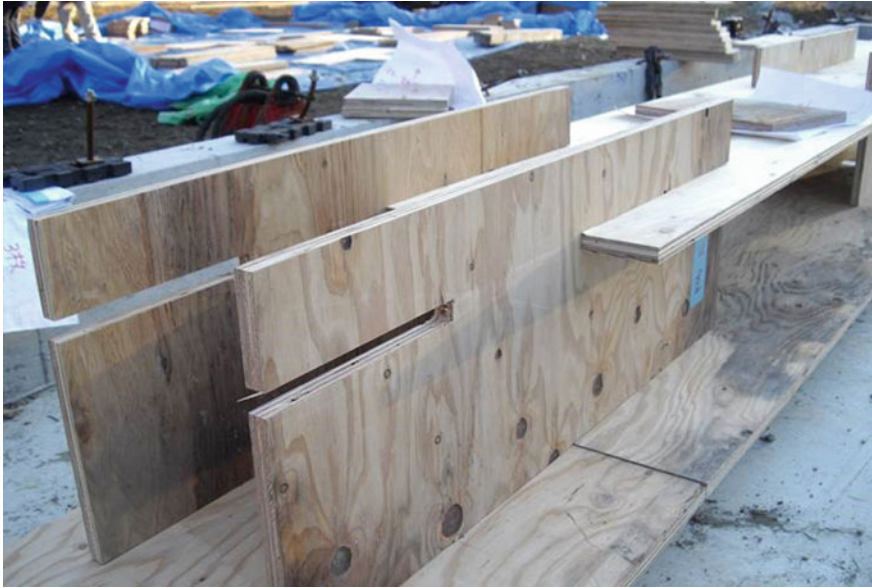
Fig. 24.2 Veneer house, notched construction system
