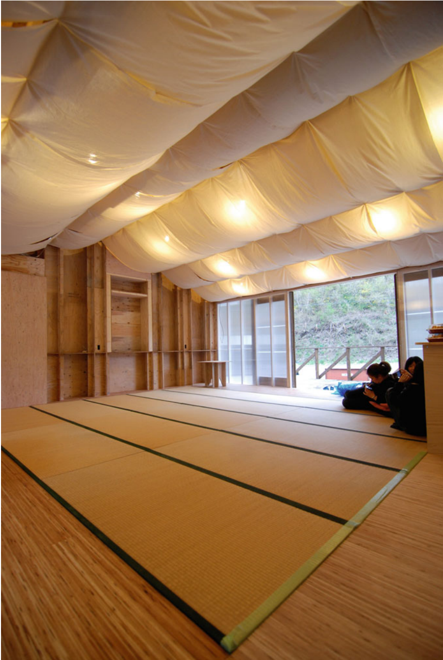
Fig. 24.5 Living space with LVL flooring
