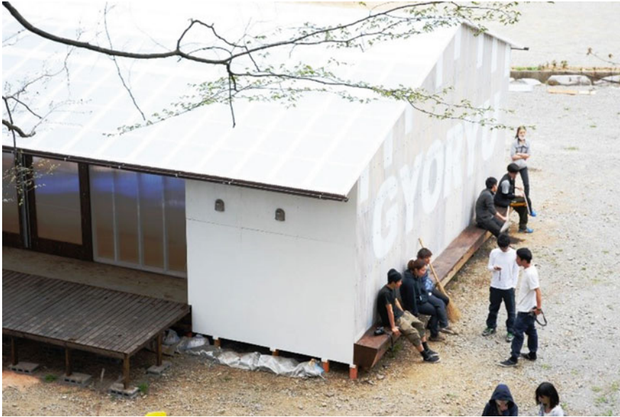
Fig. 24.3 Minami-sanriku Community House (Veneer House 1)
