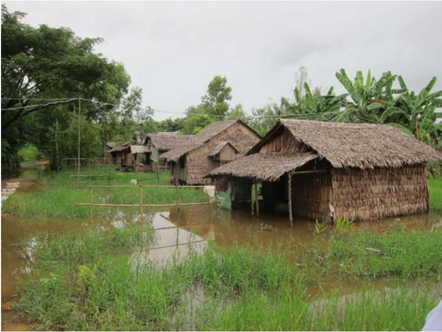
Fig. 24.10 Flooding in Myanmar overwhelms local housing
