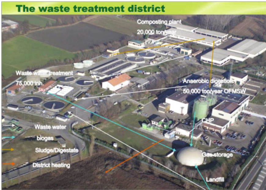
Fig. 6.1 Aerial view of Acea Pinerolese Industriale municipal waste management plant
