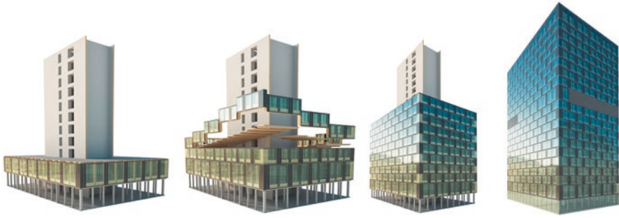
Fig. 26.2 The LCT ONE was constructed in 8 days (Source: Cree GmbH)
