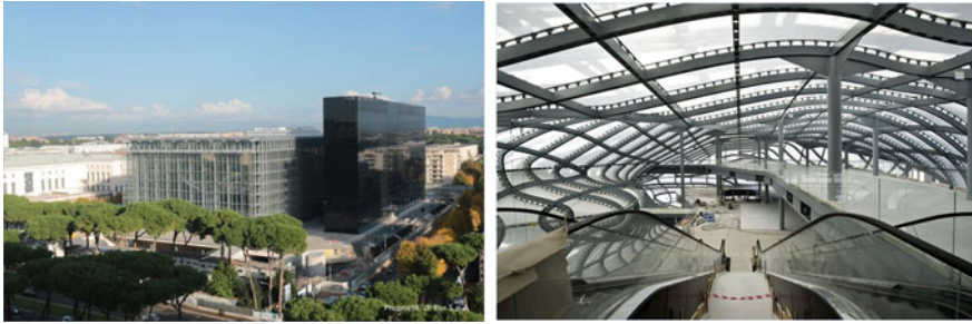
Fig. 3 The new Conference center “Nuvola” (Rome), Source EUR S.P.A
