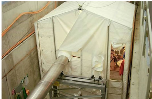
Fig. 27.26 Welding area in the tunnel
