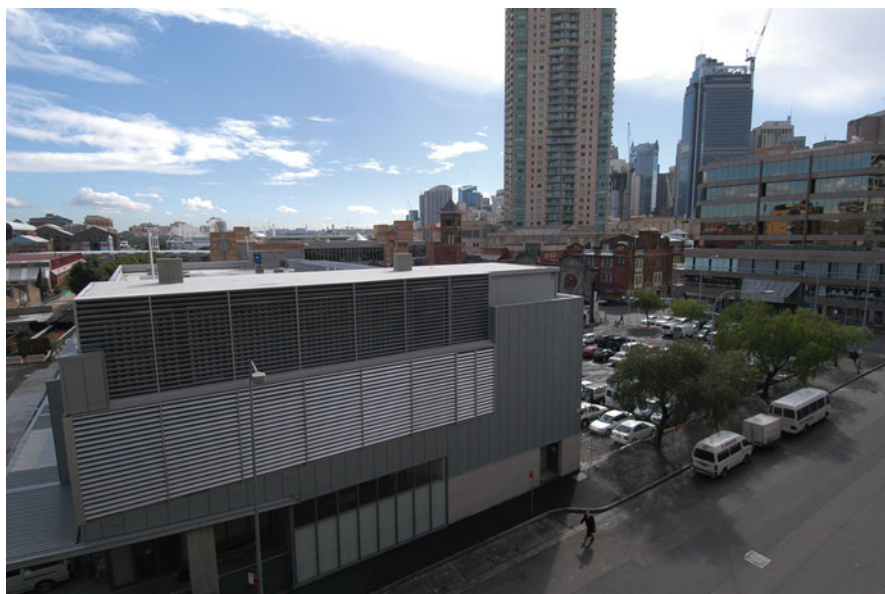
Fig. 15.6 23 bays of 145 kV GIS and 4 bays of 362 kV GIS and transformer hidden in a shopping complex
