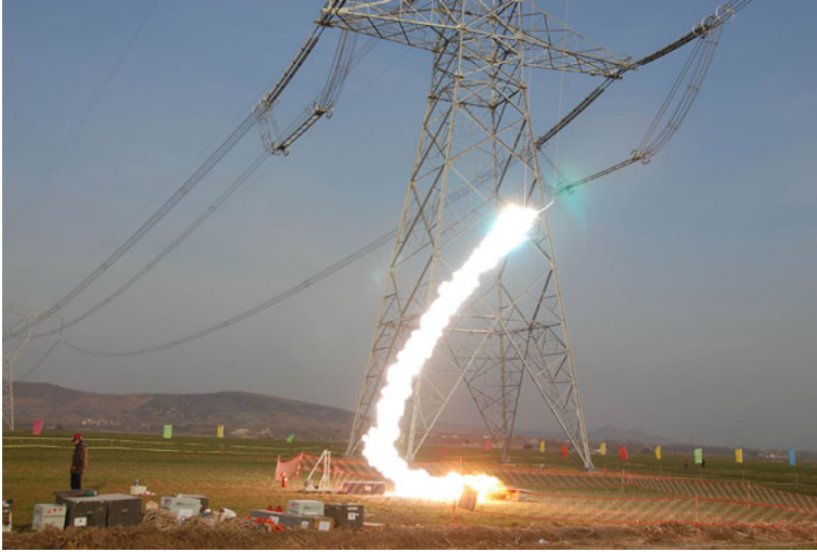
Fig. 28.4 Artificial staged fault single-phase-to-ground testing on Nanyang-Jingmen UHV line
