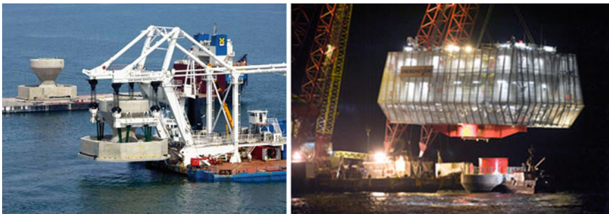
Fig. 29.27 Installation of gravity foundation. (Source: Energinet.dk)
