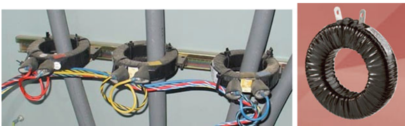
Fig. 12.19 Cable slipover current transformers and ring current transformer
