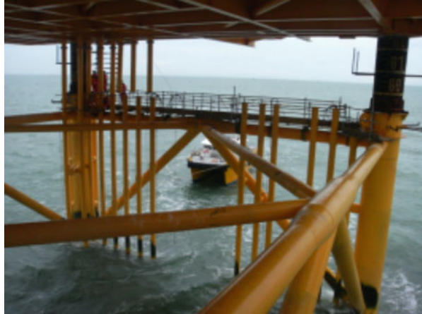
Fig. 29.22 Example of J-tube filler sections being installed between jacket and topside
