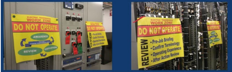
Fig. 14.5 Example of work zone identification marking
