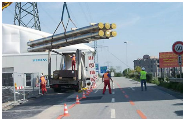
Fig. 27.24 Delivery of transport units at preassembly area
