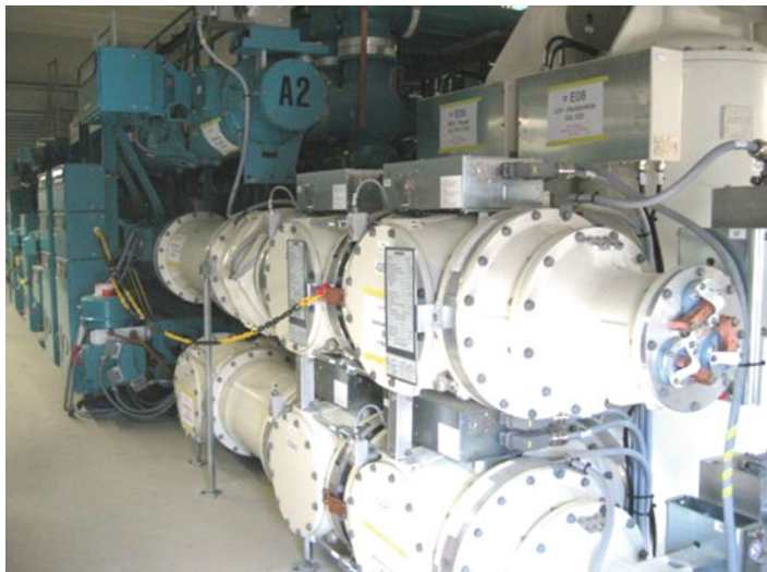
Fig. 16.2 Extension of a GIS with three-phase busbar
