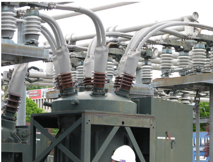
Fig. 11.51 Shielding of HV connections from animals: example from Canada (CIGRE 2016)
