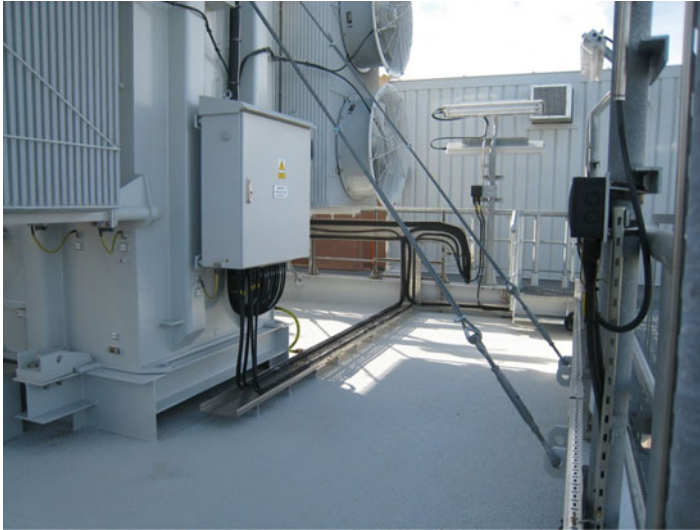
Fig. 29.16 Example of temporary bracing on a transformer for sea transportation
