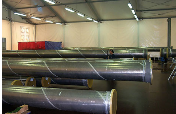
Fig. 27.25 Preassembly of GIL sections
