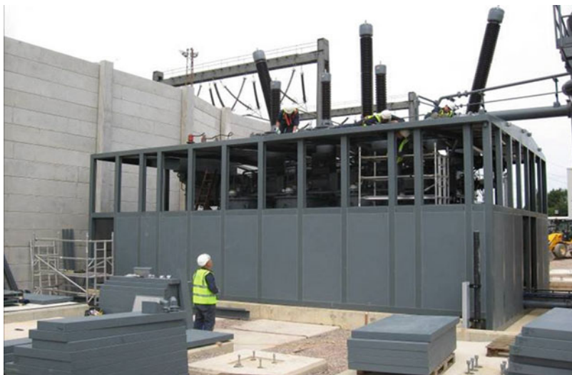
Fig. 12.50 Acoustic enclosure under construction
