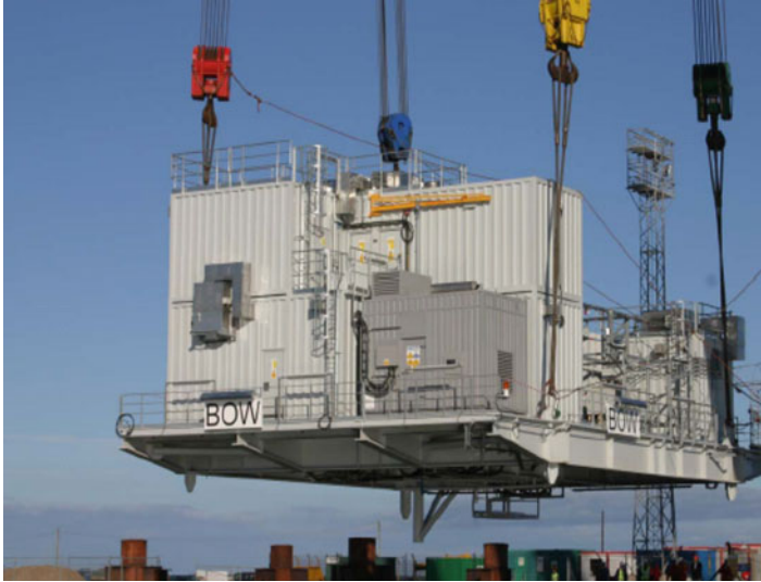
Fig. 29.12 Enclosure of containerized offshore substation
