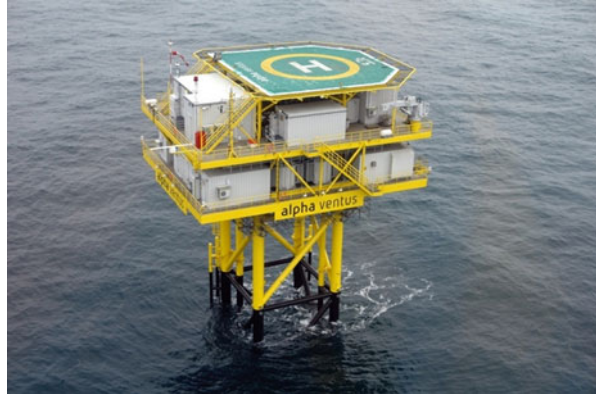
Fig. 29.24 Topside with two container decks. (Source: ALSTOM Grid GmbH)
