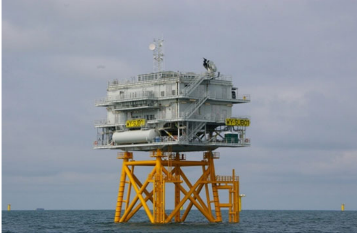
Fig. 29.26 Jacket substructure: Walney 1. (Source: DONG Energy)
