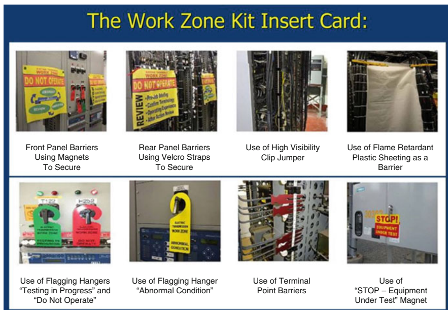
Fig. 14.6 Example of work zone identification marking
