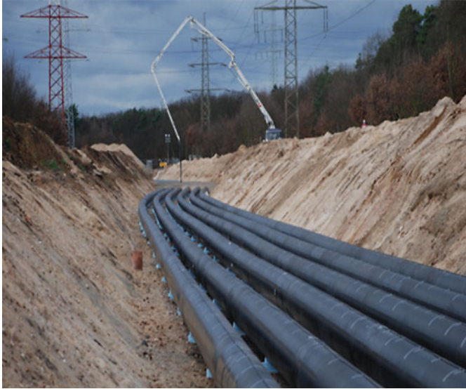
Fig. 27.18 Six single-phase GIL pipes in the trench before backfilling
