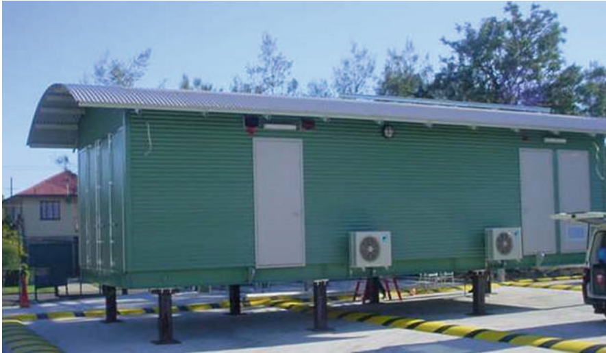
Fig. 6.7 Example of a prefabricated substation for permanent installation on-site. (Courtesy Ergon Energy, Australia)
