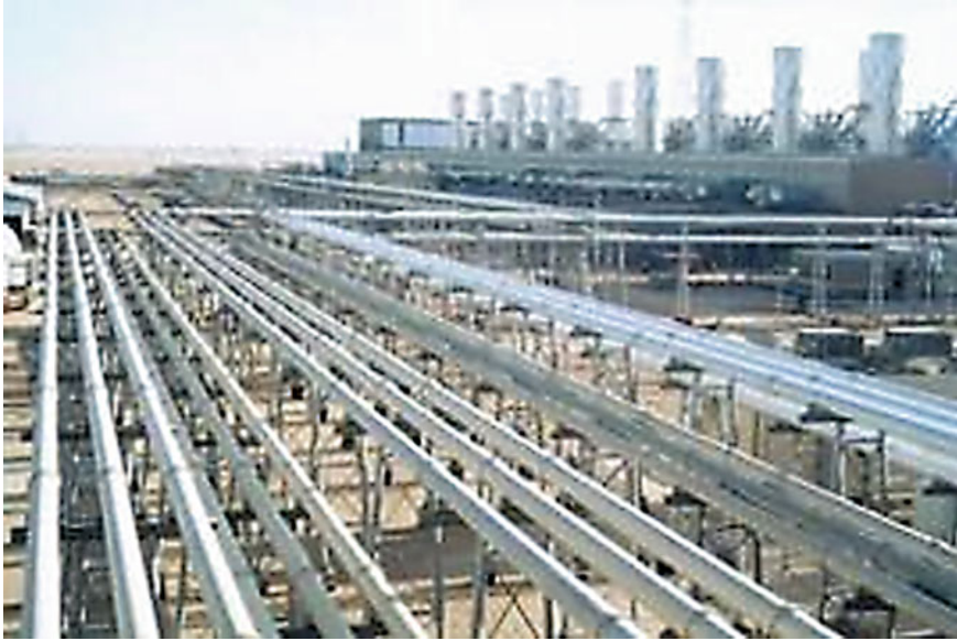
Fig. 27.12 Views of the 420 kV PP9 GIL: erection and layout
