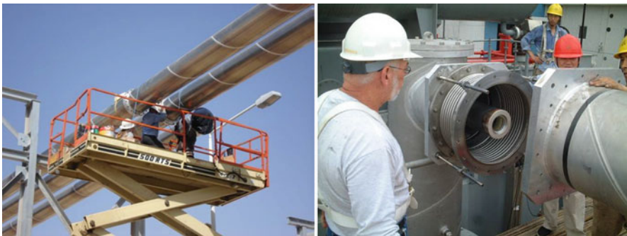
Fig. 27.31 Installation of section of bus bar on-site
