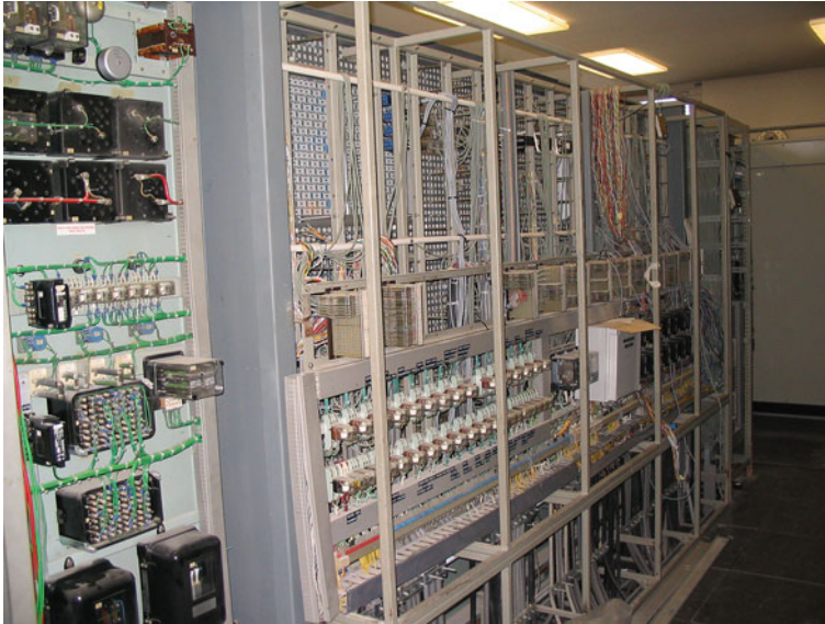
Fig. 53.1 Existing protection panels
