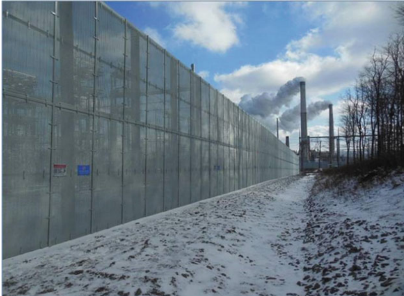
Fig. 11.50 Example from America of security fencing to provide some protection against vandalism from firearms
