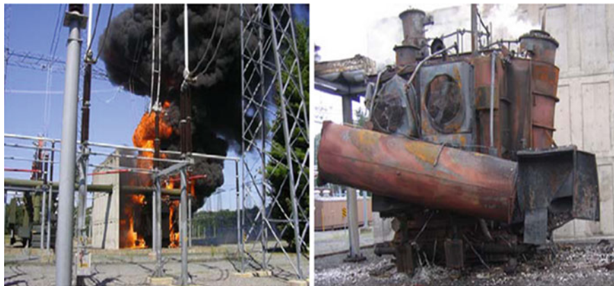
Fig. 51.1 Examples of catastrophic failures of substation equipment (CIGRE 2011)
