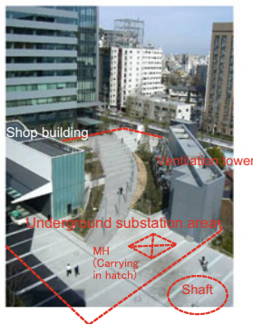
Fig. 20.2 Indoor and underground mixed substation (Chubu Electricity Company, Inc. Ushijima-Cho S/S)
