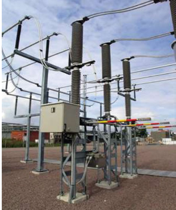
Fig. 26.7 Combined switchgear – circuit breakers, disconnectors, and earthing switches (ABB Catalogue)
