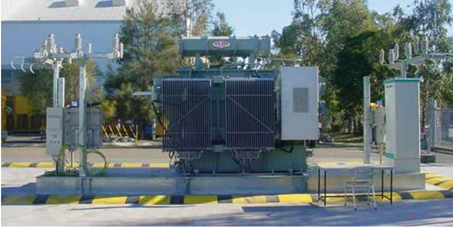
Fig. 6.6 Skid mount substation (courtesy Ergon Energy, Australia)
