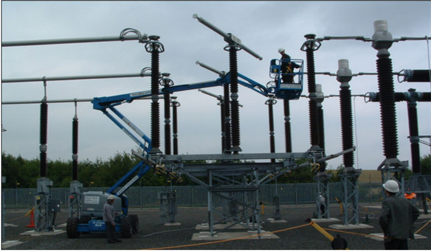
Fig. 5.7 Example of a MEWP being used to carry out maintenance work
