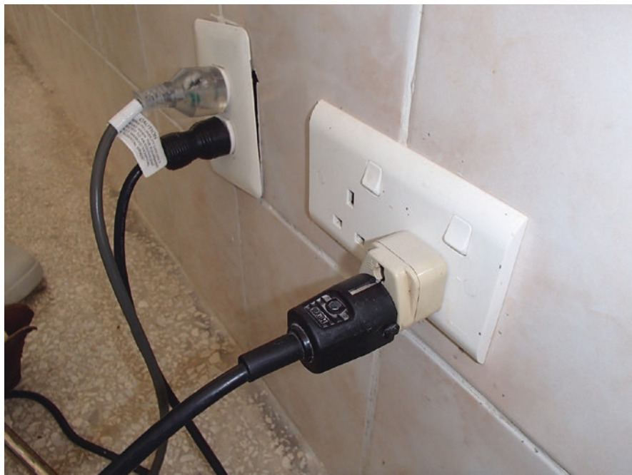
Fig. 10.4 Power outlets will vary not only in styles but in voltage and frequency. Always make sure the device is plugged in to the correct power source
