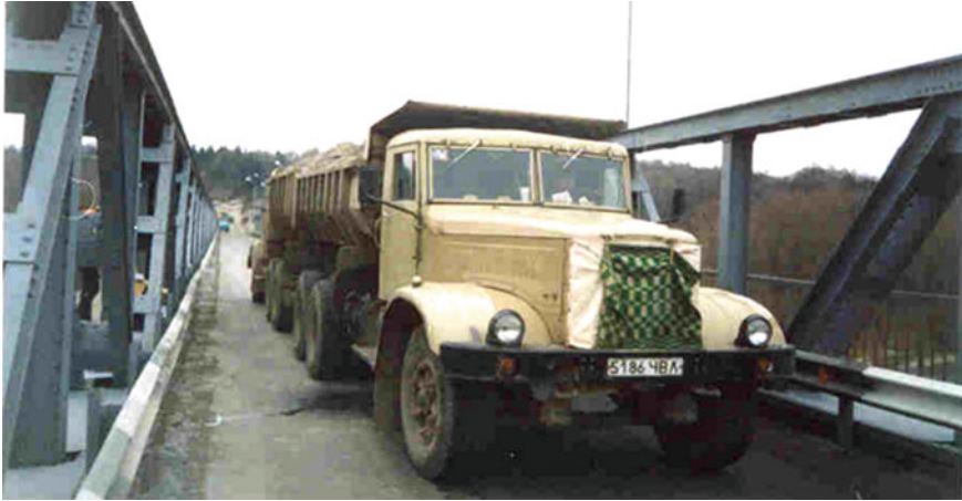
Fig. 6.31 Loading the bridge span 1–2 by two “KrAZ” tipper trucks
