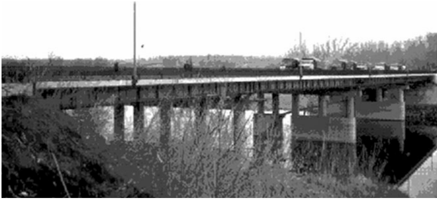
Fig. 6.27 General view of the bridge during testing
