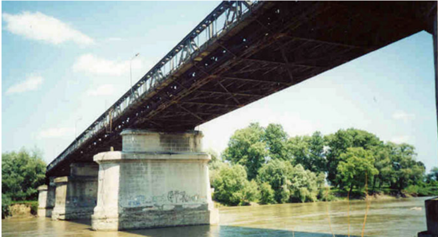
Fig. 6.30 A general view of the bridge across the Prut River in Chernivtsi
