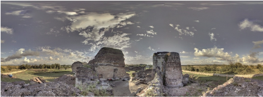
Fig. 3. 360° spherical photo: general view on the palace
