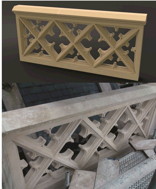
Fig. 2. Balustrade for the St Martin’s basilica in Halle (Flanders, Belgium), which has been cut out of stone, using a digital model created by CAD (© Visuaxis)
