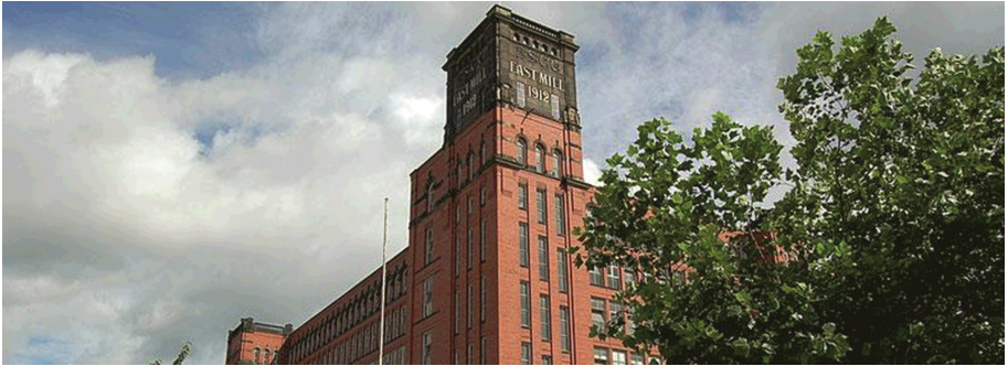
Fig. 4. Derwent Valley Mills, UK
