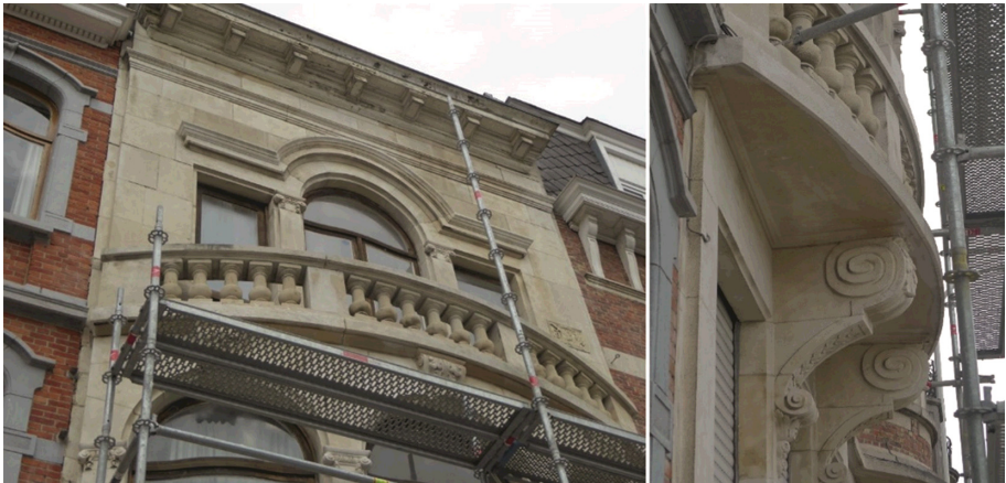
Fig. 4. An example of historic architecture (Leuven, Flanders) that turns out to be constructed entirely of ‘artificial’ natural stone, during the reconstruction period after the First World War (around 1920), illustrating the fact that application of artificial stone in itself is not new at all. With the naked eye, this ‘concrete’ is hardly distinguishable from actual natural stone.
