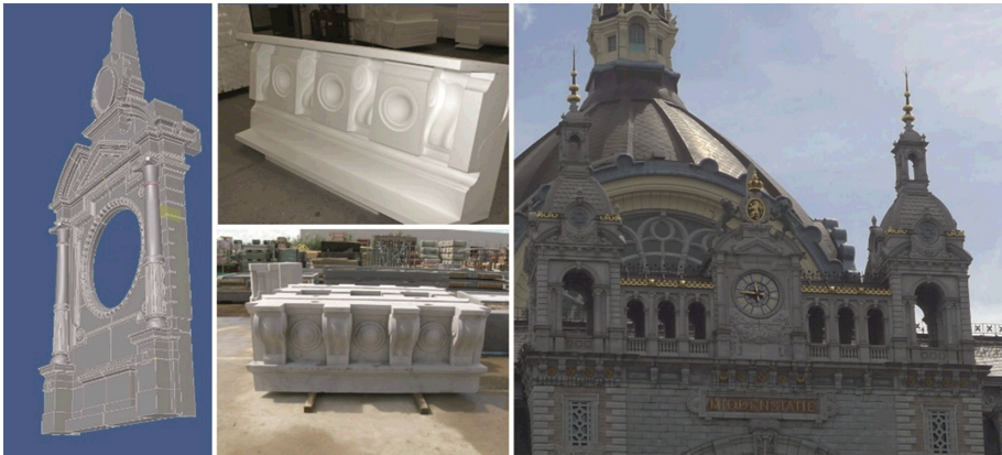
Fig. 5. Different stages in the reconstruction of the clock-pavilion of the Antwerp Central Station. From left to right: part of the digital model of the clock-pavilion (© Verstraete&Vanhecke), the EPS-mold and the cast model (©Twinplast), the completed clock-pavilion.
