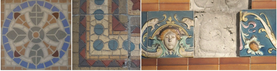
Fig. 7. Different types of ceramic tiles that may benefit from developments in the 3d-printing technology. Quite often one tries to find such tiles in antiques shops (which quite often works out well). In some cases such tiles need to be reproduced. For the two tiles on the left (a flat floor tile, and a tile with a surface relief) the technology is readily available to 3d-print the mold (several materials are available, and one can print the mold taking into account the shrinkage of the clay while cooking). This is not yet the case for the type of tiles in the right image, further research is necessary.
