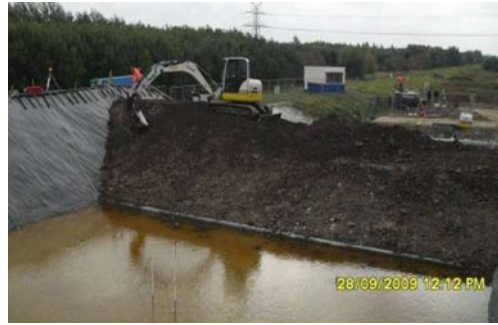
Fig. 4 Levee construction in the IJkdijk large-scale test #2 [32]
