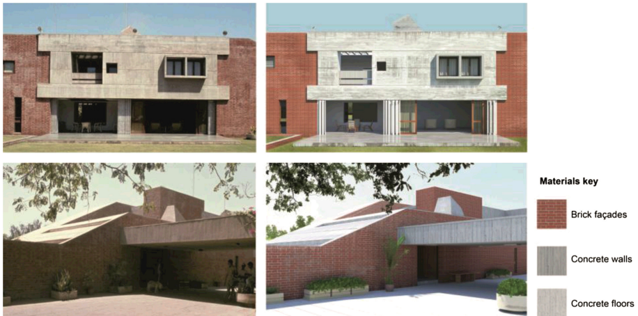
Fig. 4. Ramkrishna House in Ahmedabad, by Chalres Correa: original pictures (left side) and photo-realistic views (right side). Rendering by E. Ranuzzini, O. Ballardini, D. Felloni.
