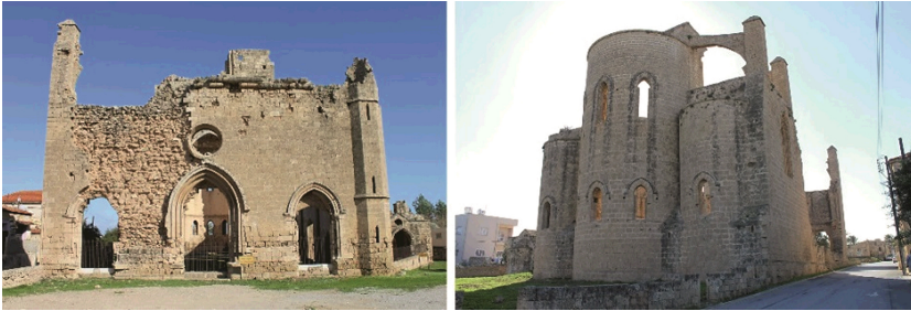
Fig. 1. Left - the West end of the Cathedral of St George of the Greeks showing the rose window/oculus. Right - the East end of the Cathedral showing the three apses, lancet windows and flying buttresses supporting the clerestory.
