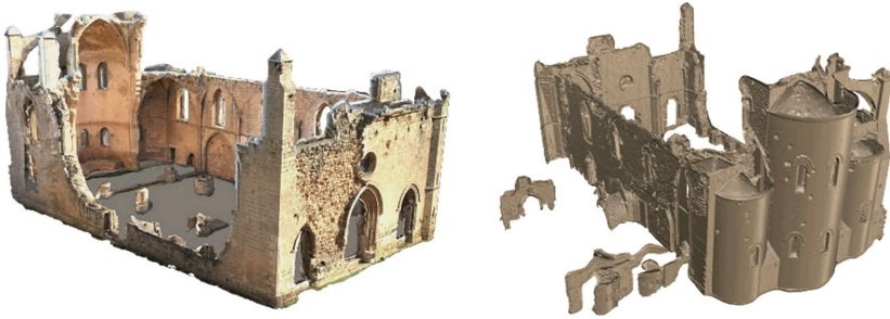
Fig. 2. Left – the 3D digital model of the Cathedral as it exists from the North West showing the photo-textures overlaid upon the surface of the geometric model. Right – the 3D digital model without photo-textures, viewed from the south east.
