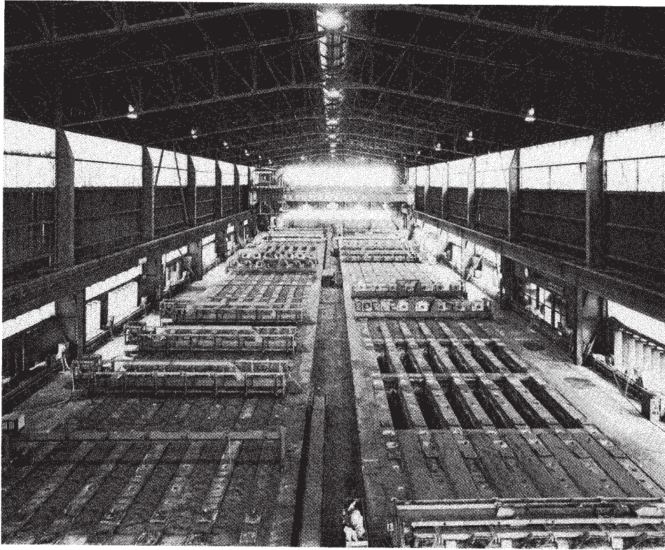
figure 1: Open ring-type bake furnace
