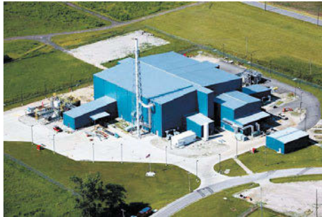
Figure 9 – New Materion “Pebbles Plant” located in Elmore, Ohio, USA.
