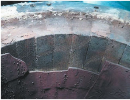
Figure 7: Ring 5 With Portion of Frozen Slag Layer Removed
