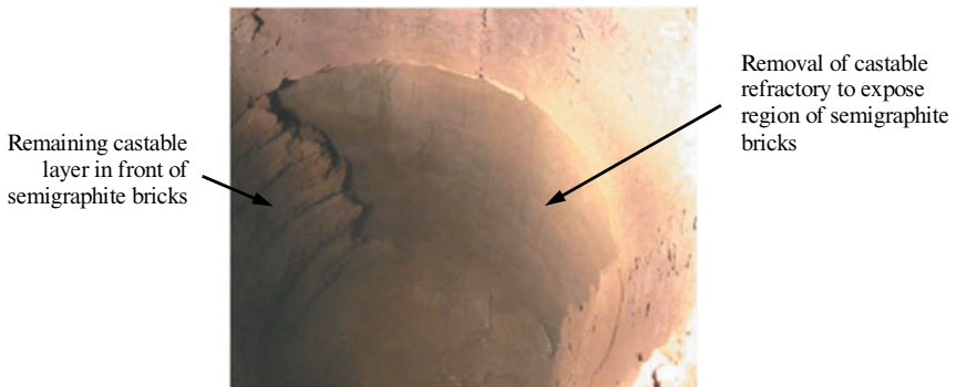
Figure 5: Section of Castable Refractory Removed Prior to Trial 3
