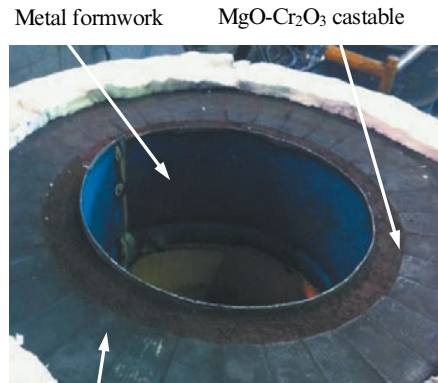
Semigraphite lower wall bricks (Ring 5)
