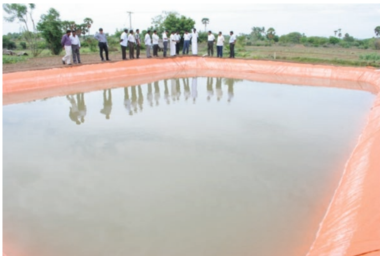
Fig. 1 HDPE-lined farm pond at Namakkal, Tamil Nadu
