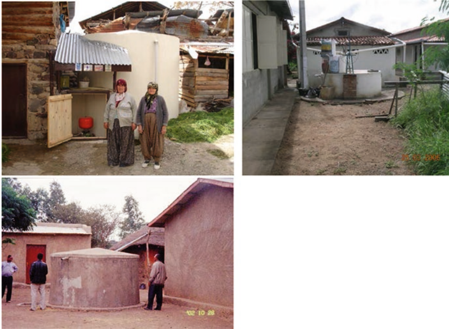
Fig. 3 Rooftop water harvesting in Bey pazari in Turkey (top left), Brazil (top right) and Ethiopia (bottom) (Source: Akhtar Ali personal communication)
