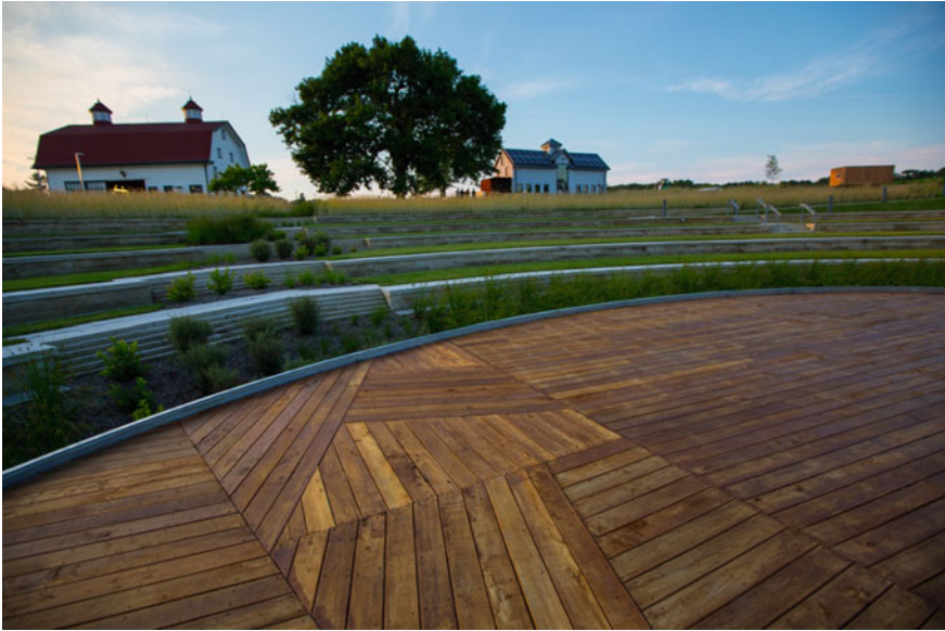
Fig. 1 View of existing barns from the main stage of the Amphitheatre; an outdoor gathering space designed as part of the phase 1 campus development; the Dairy Barn on the right has been renovated into a campus cafe
